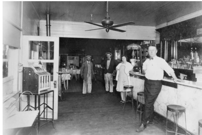
Image of the inside of a restaurant near Maxwell, California, ca. 1927 Source: Sacramento Valley Museum.
