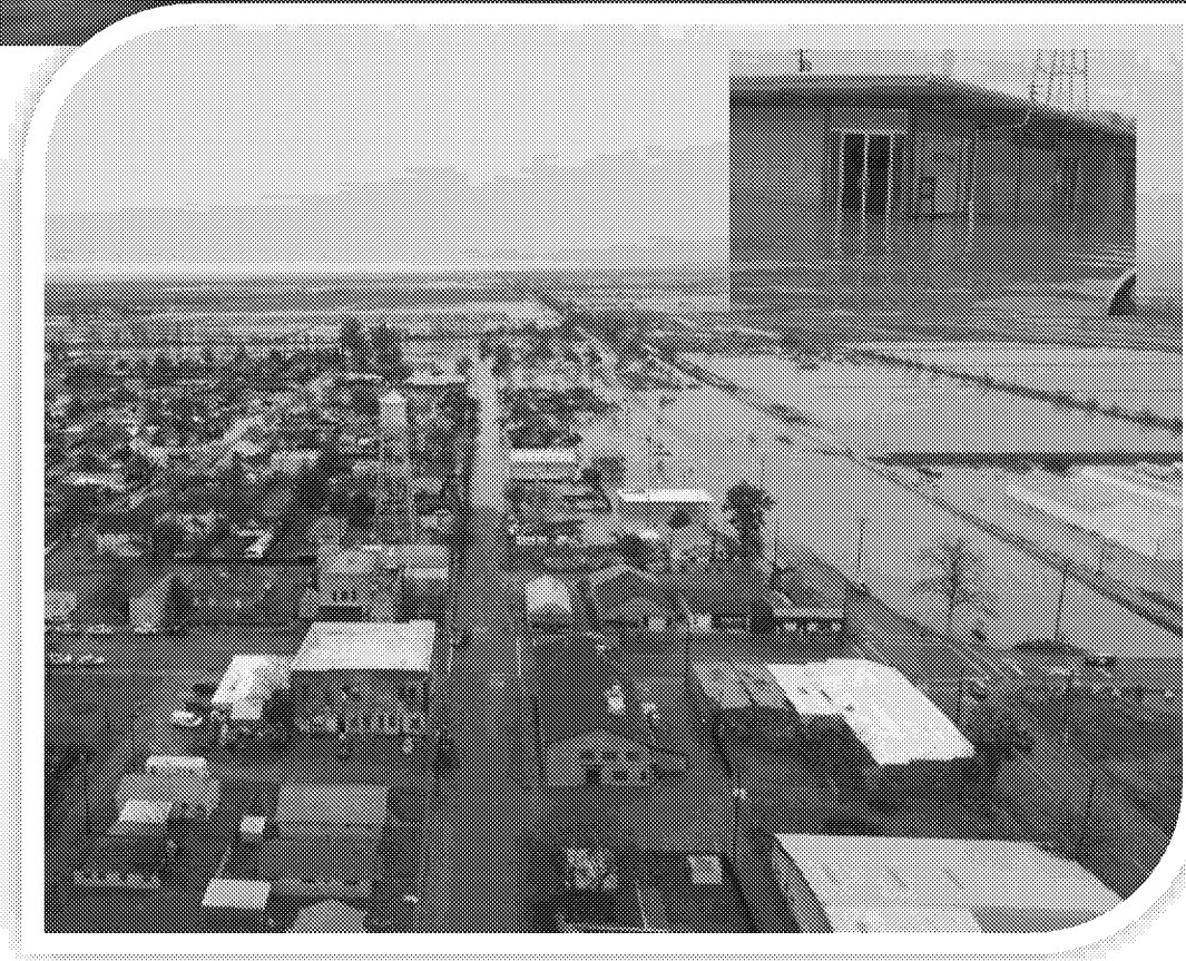
Flooding in Maxwell, CA in Feb 2017
