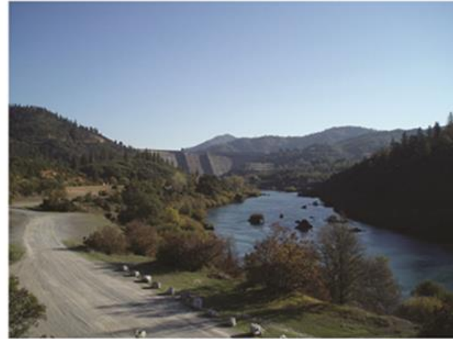
Shasta Dam VAU, KOP 9, Photo 9a View from the road above the Chappie - Shasta OHV Area staging area looking northeast.
