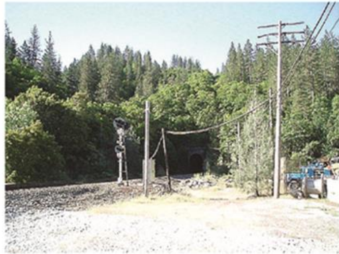
Bridge Bay VAU, KOP 3, Photo 3a View of the Union Pacific Railroad train tunnel looking south from the Bridge Bay Resort maintenance area.
