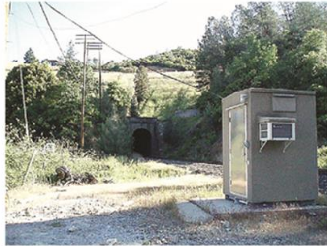
Bridge Bay VAU, KOP 3, Photo 3b View of the Union Pacific Railroad train tunnel looking north from the Bridge Bay Resort maintenance area.
