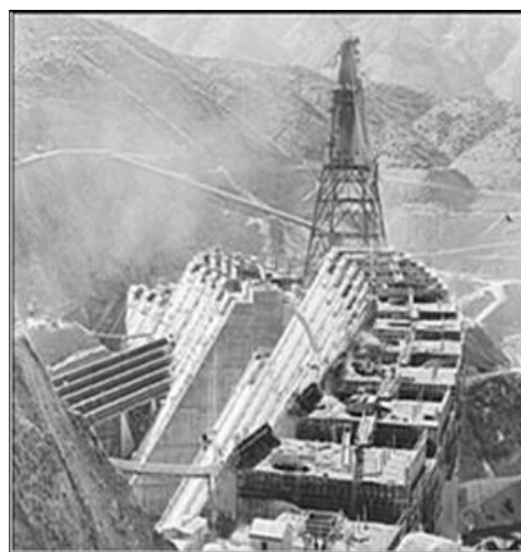
Shasta Dam Under Construction
