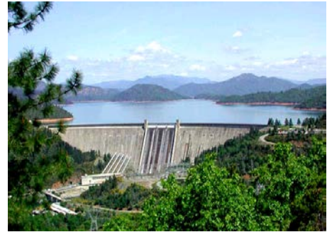
Present Shasta Dam
