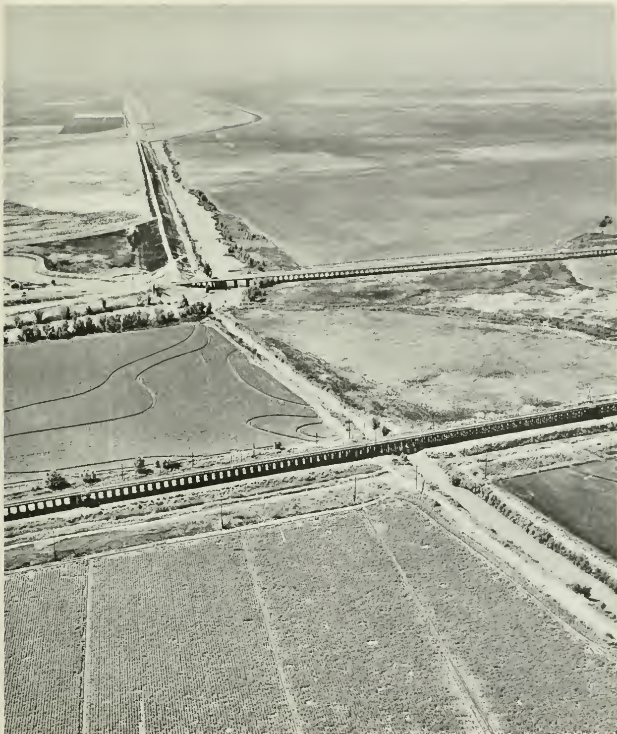
View of Tule Canal looking southward showing restricted channel capacity above Highway 40 crossing. Sacramento Deep Water Ship Channel and toe drain can be seen in background.
