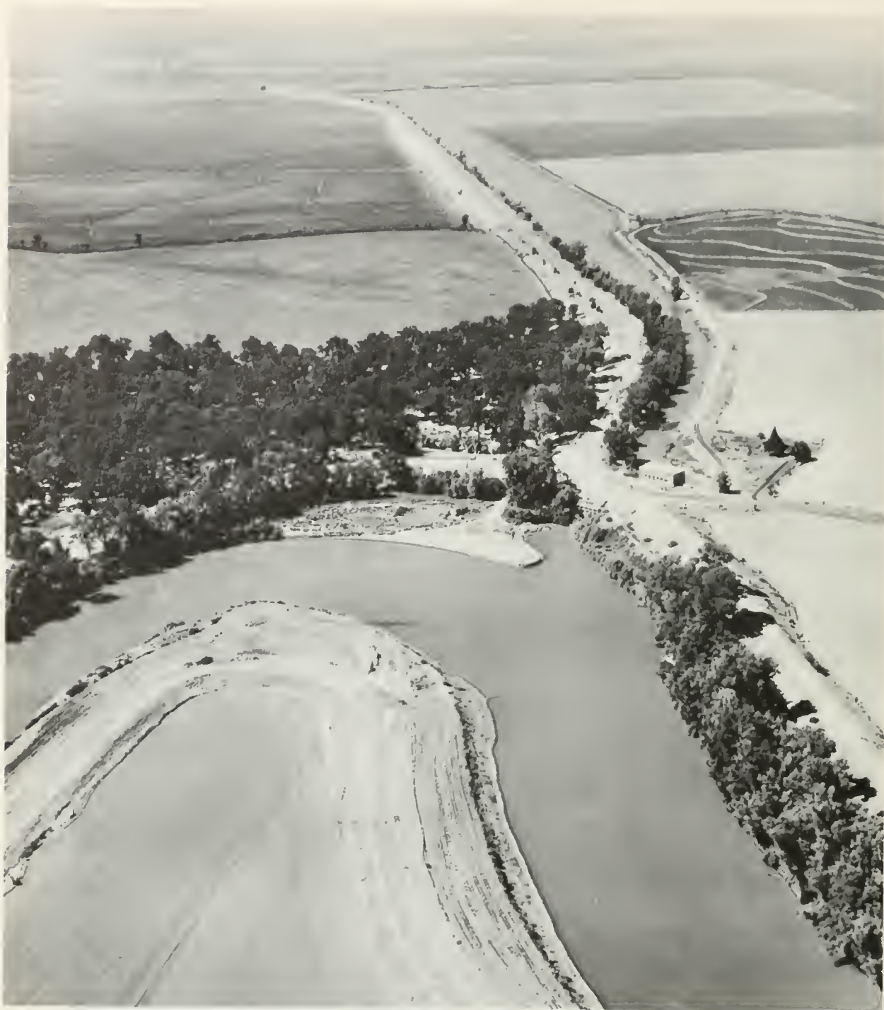
A pumping plant on a branch of the Colusa Basin Drainage Canal was originally constructed to pump flood waters into the Sacramento River. However, it is not used for flood relief, but supplies irrigation water to lands in the Colusa Basin.
