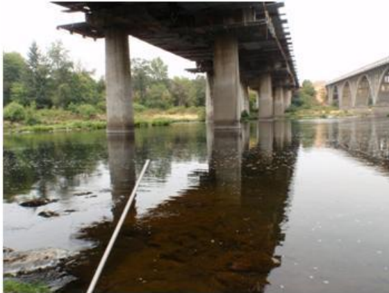
Photo 1: 7/31/2009 (by the highway piling)
