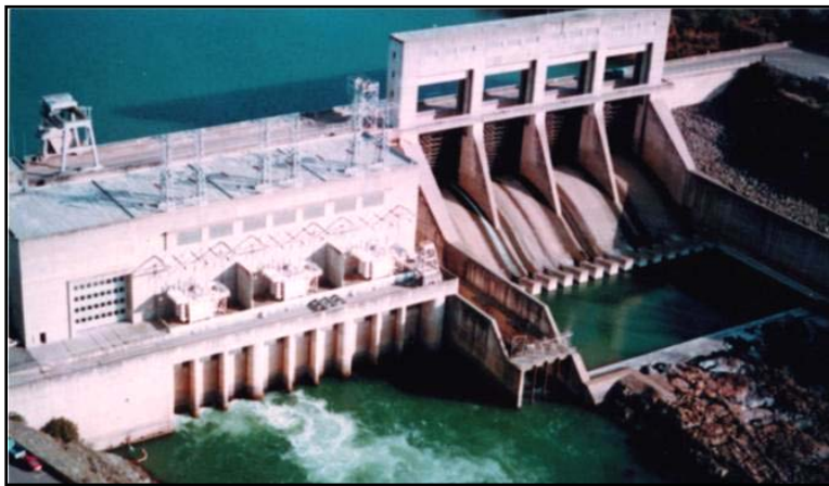
Figure 13. Keswick Dam located at river mile 302 on the upper Sacramento River. The stilling basin on the right side of the picture used to trap adult anadromous salmonids. Aerial photo by Dave Vogel.
