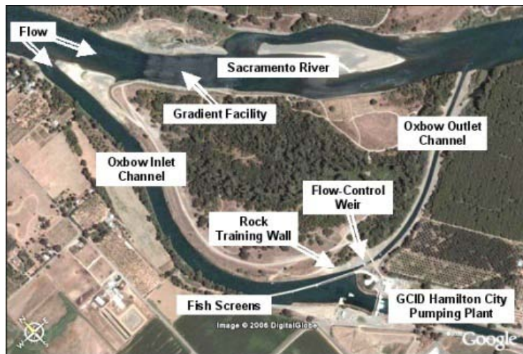
Figure 35. Aerial view of the new GCID fish screens and gradient facility on the Sacramento River near Hamilton City (from Vogel 2008a).
