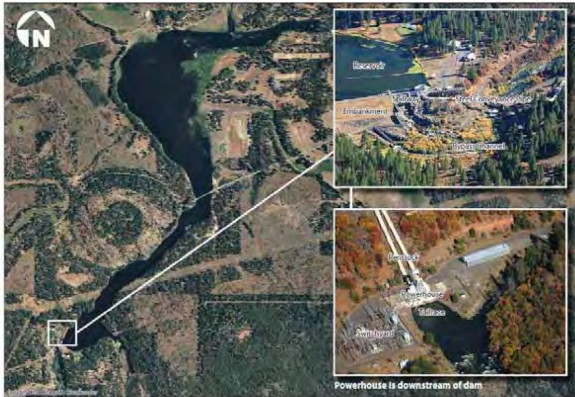
Figure 3.19-9. View of J.C. Boyle Powerhouse.
