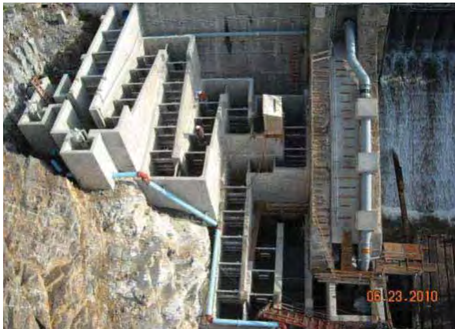
Figure 3.19-11. Example of fish ladder built into steep bedrock similar to Copco 1 option (photo courtesy of GEI Consultants).
