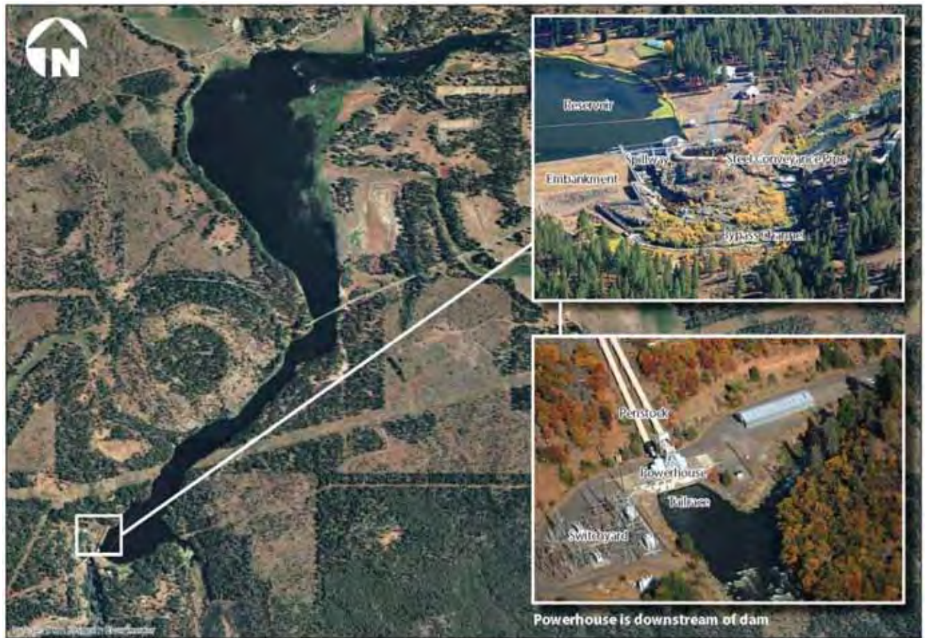
Figure 2-2. J.C. Boyle Dam and Powerhouse.
