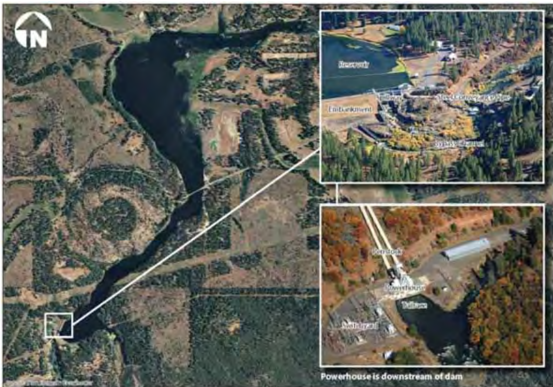
Figure ES-3. J.C. Boyle Dam and Powerhouse.
