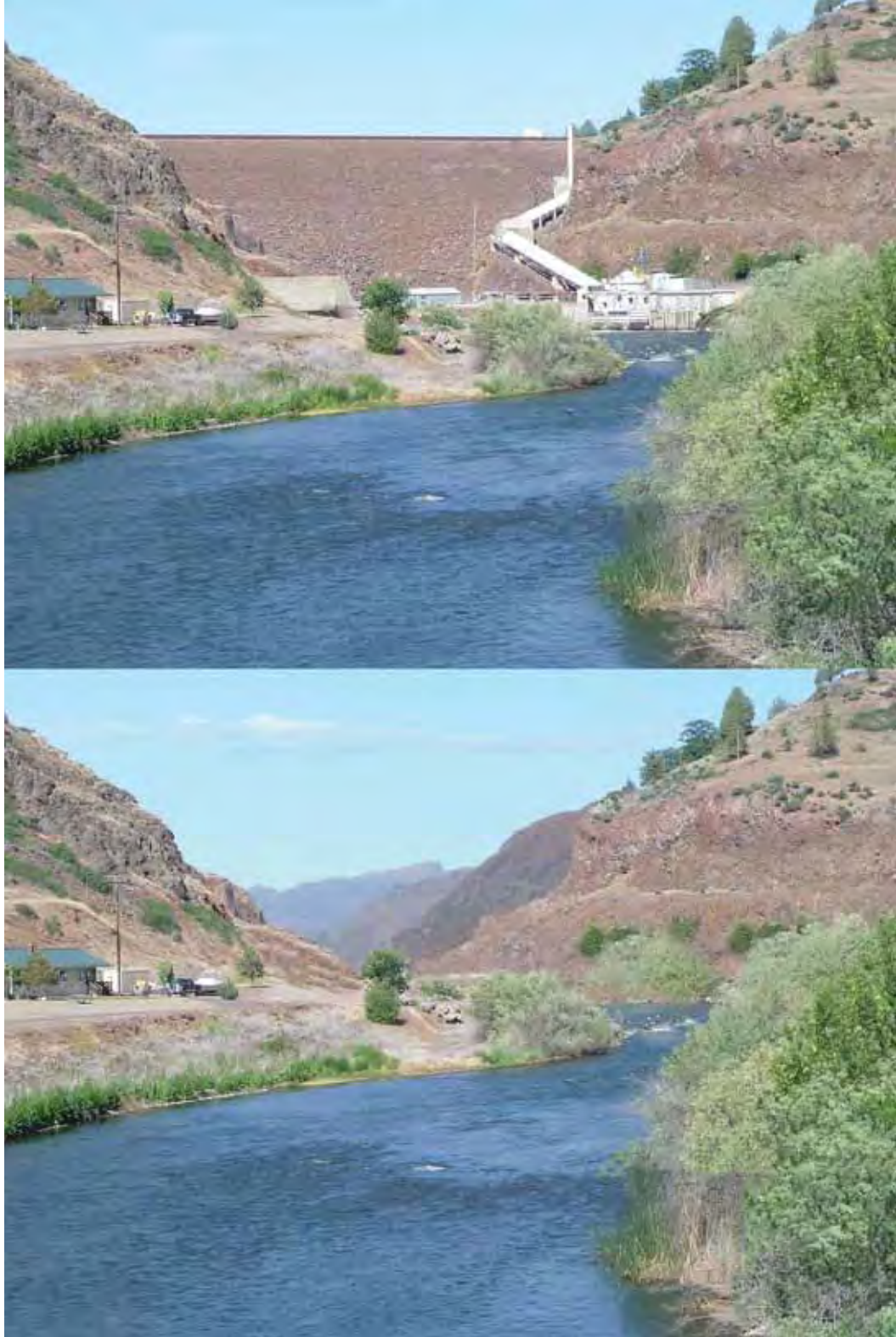
Figure 3.19-6. Iron Gate Dam before removal (top) and a simulation of what the facility could look like after full removal (bottom) except for Landform/Vegetation restoration details which cannot be fully depicted until completion of the Definite Plan.
