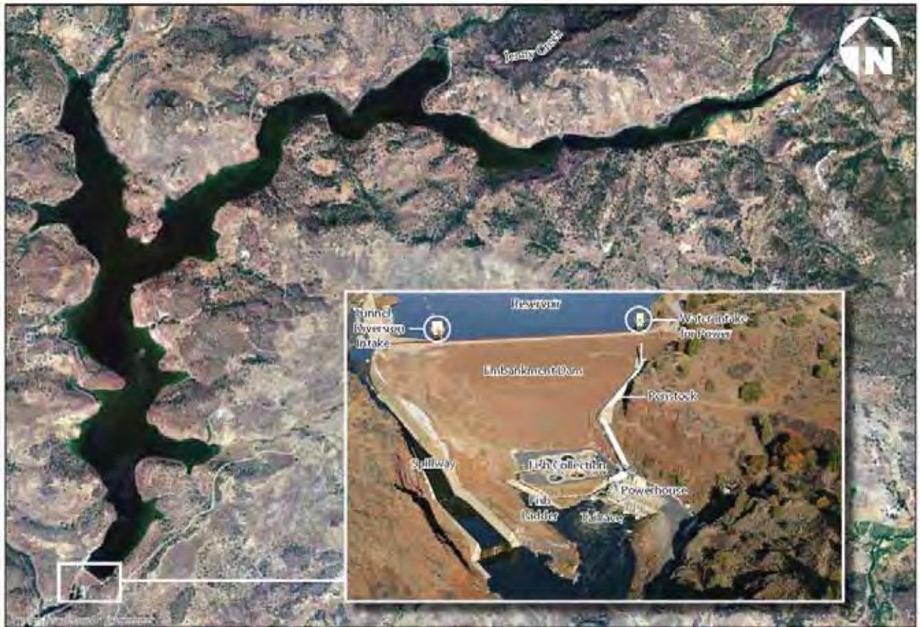
Figure 2-6. Iron Gate Dam, Reservoir, and Power Generating Facilities.
