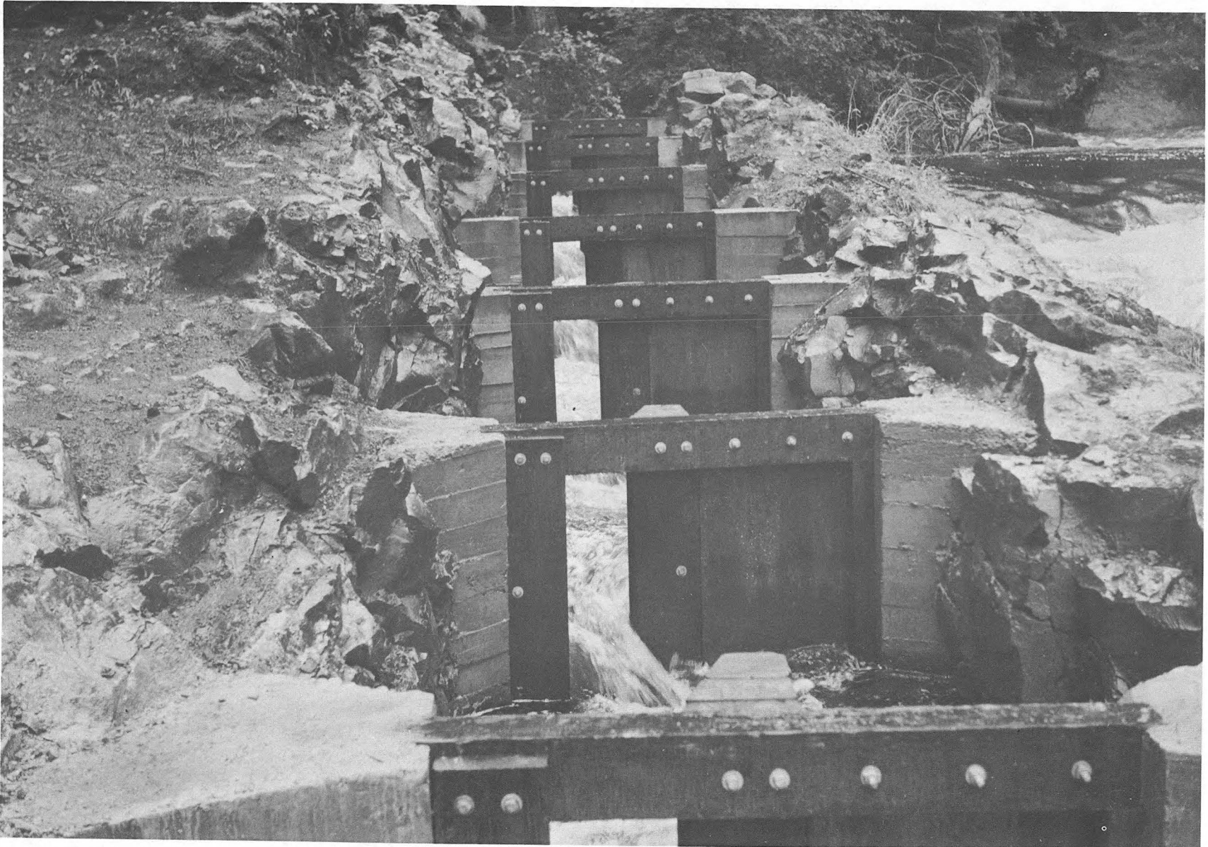
SLOTTED FISHWAY (WOODEN BAFFLES) Queen Charlotte Islands, British Columbia Canada Department of Fisheries
