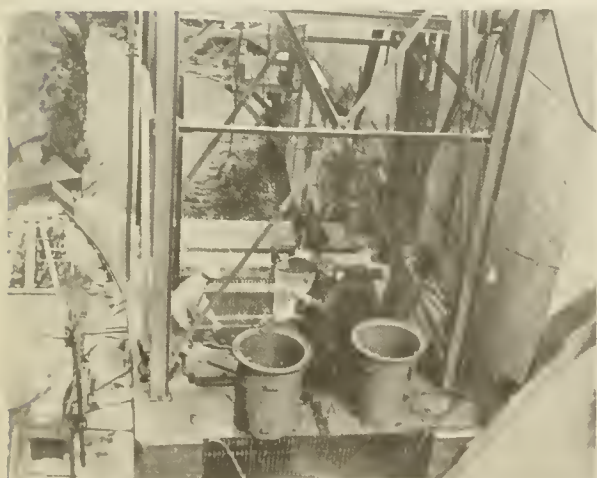
Figure 32.--Dip netting shad from trap to buckets for hoisting fish to fish-lift flume, Hadley Falls Dam, Connecticut River, Holyoke, Mass.
