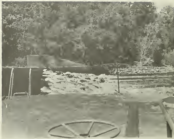
Figure 30.--Ineffective fishway on a lock and dam, Cape Fear River, N.C. The structure is on the far river shore, and little if any water passes through the transportation chamber during the months adult shad would be present.
