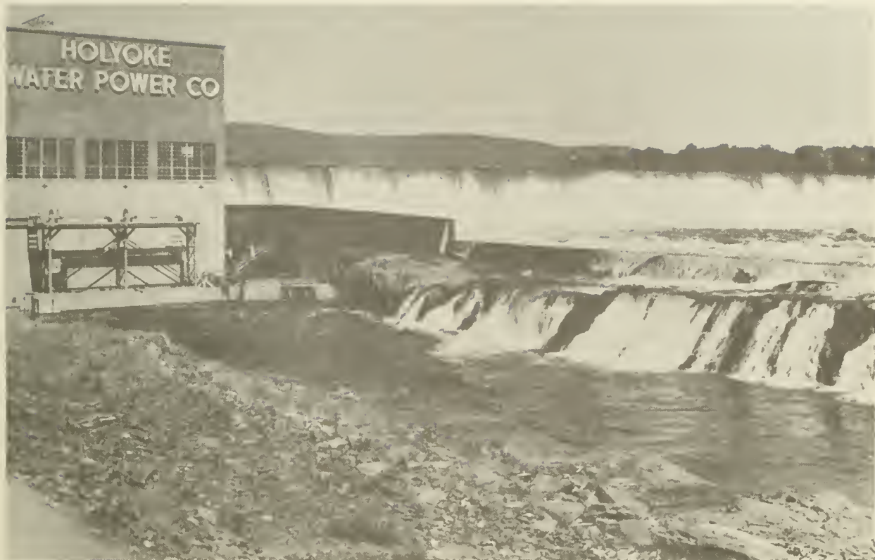
Figure 31.--Hadley Falls Dam, Connecticut River, Holyoke, Mass. Entrance and fish attraction channel on right of power plant tailrace.
