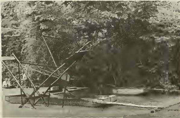
Figure 14.--Fishwheel operated on the Roanoke River, N.C. (The wire scoop revolves with the axle and captures fish in the water between the boats as it emerges from the water and dumps them into chutes leading to the boats.)
