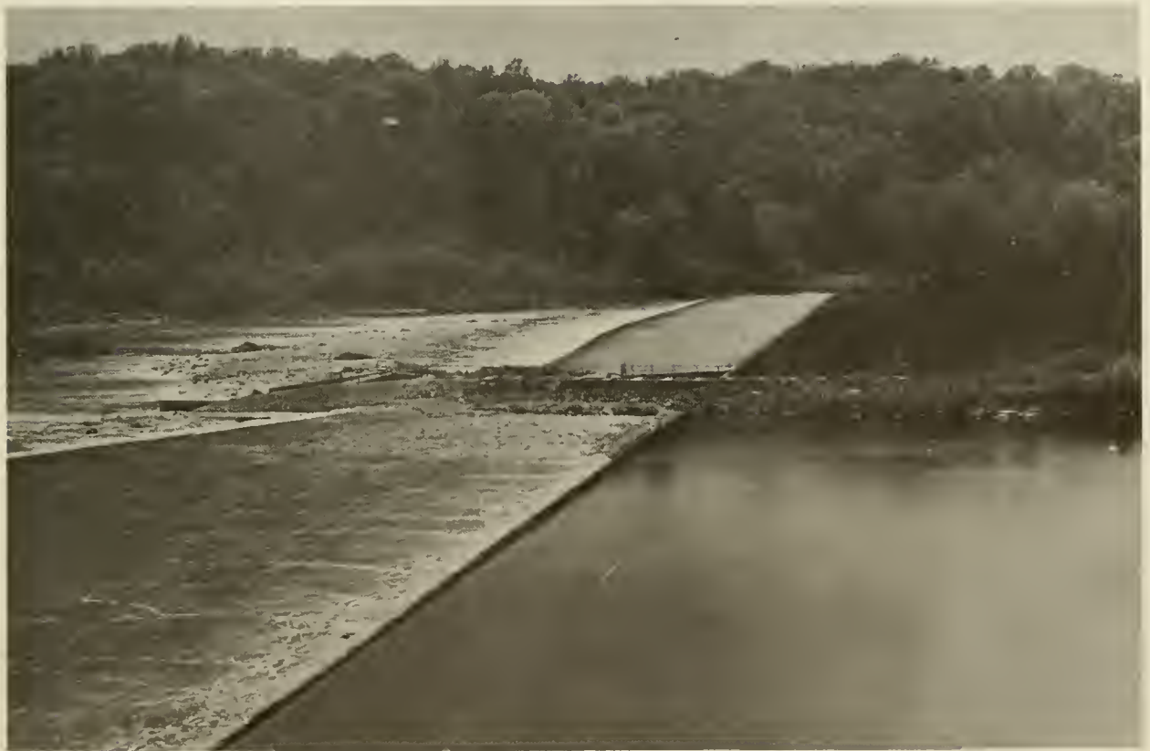
Figure 21.--Little Falls Dam, Potomac River, Md. Fishway between dams was completed in 1959.
