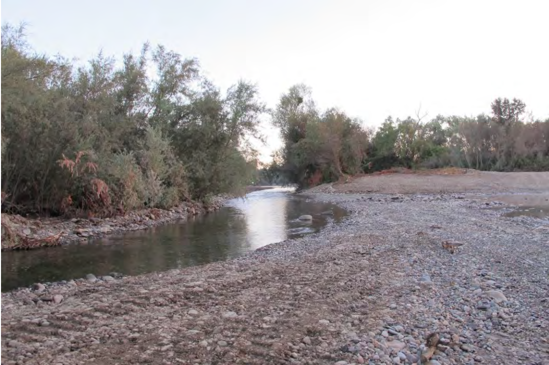
Figure 1. Side channel and restored floodplain looking northeast. Approximately 4.5-6 feet of materials were removed to lower gradient to increase amount of juvenile salmon rearing habitat over a wider range of flows.
