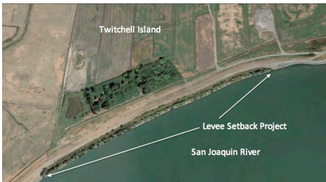
Figure 8. The Twitchell Island setback levee project is located along the lower San Joaquin River on the south side of Twitchell Island at the center of the photo. It consists of a small tidal channel and island connected at several locations with the river.
