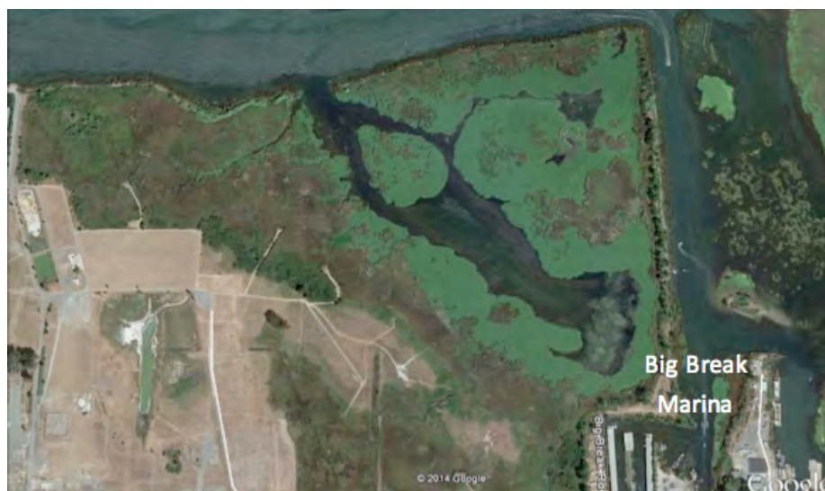
Figure 6. The west end of Big Break is a failed chemical company mitigation site. Some of the chemical waste facilities can be seen at the lower left. The site is virtually abandoned. Big Break Marina is located at the right.
