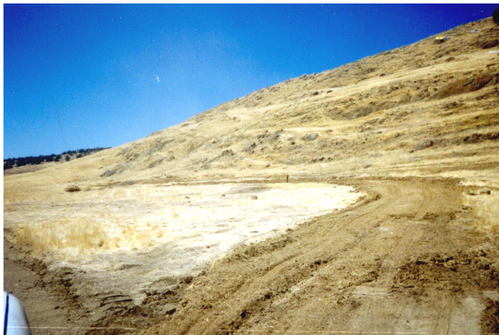
Photo 26. Site of proposed northernmost spillway at Golden Gate Inlet-Outlet Works
