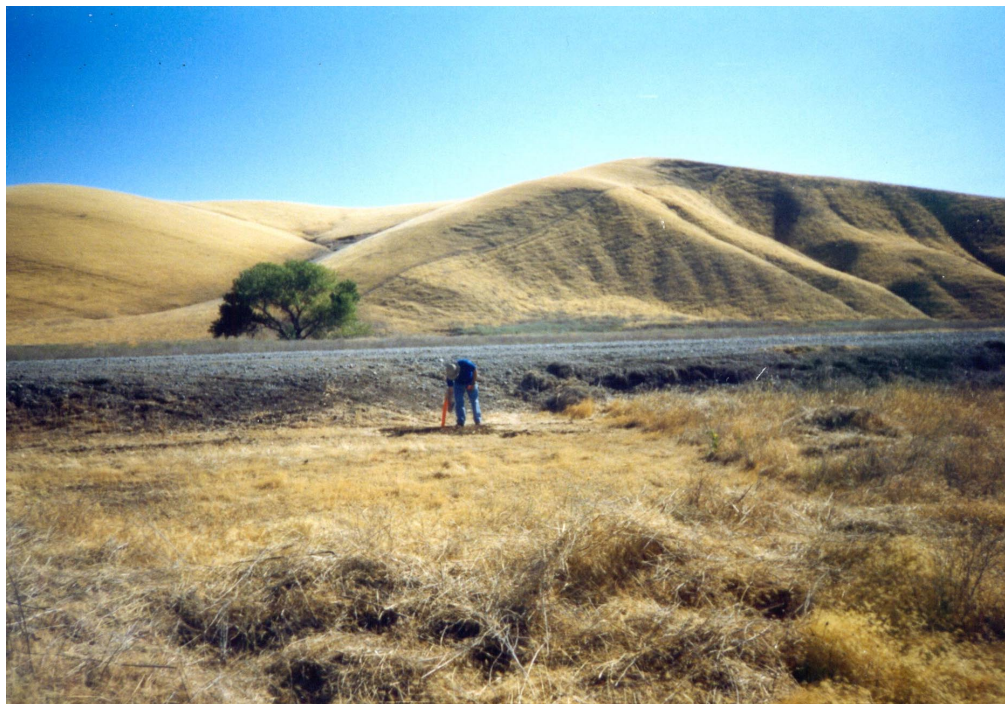
Photo 24. Site preparation at approach channel auger hole AUG-2
