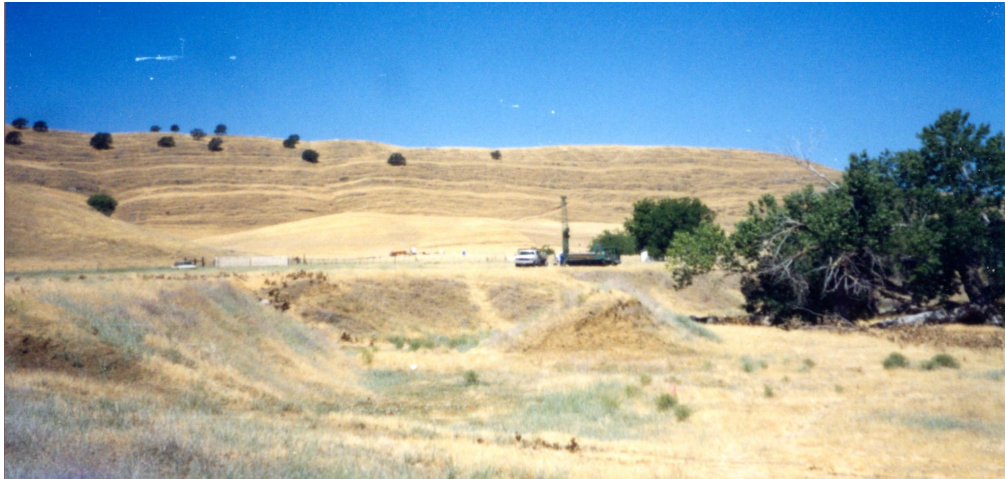
Photo 25. CME-850 drill rig at approach channel auger hole AUG-3
