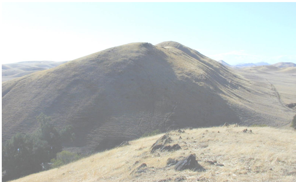
Photo 44. Southern view of right abutment of Logan Dam site
