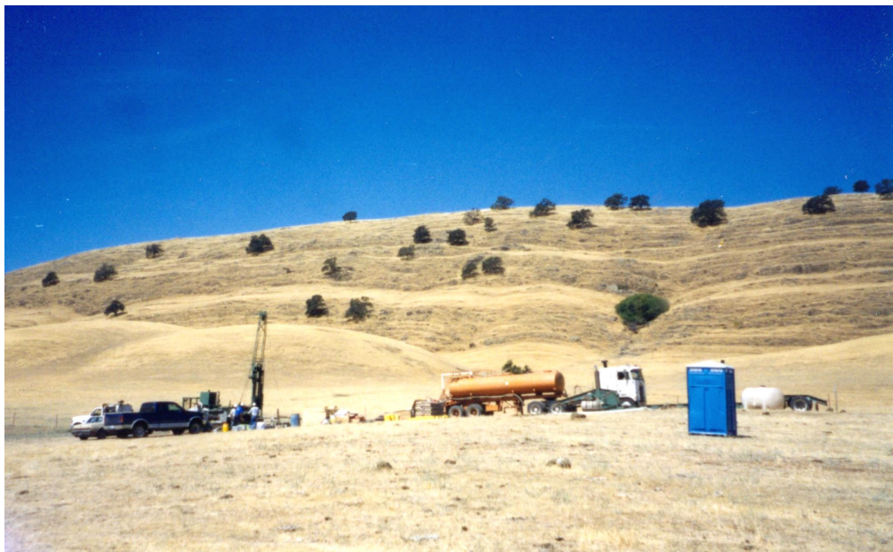
Photo 23. CME-850 drill rig at pumping plant drill hole DHPP-1
