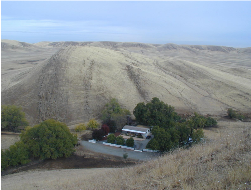
Photo 43. Northern view of left abutment and channel of Logan Dam site
