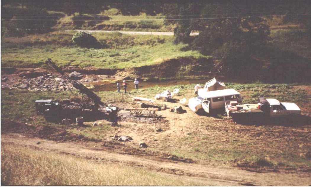
Photo 4. CME - 850 drill rig at Sites Dam site drill hole LC-2
