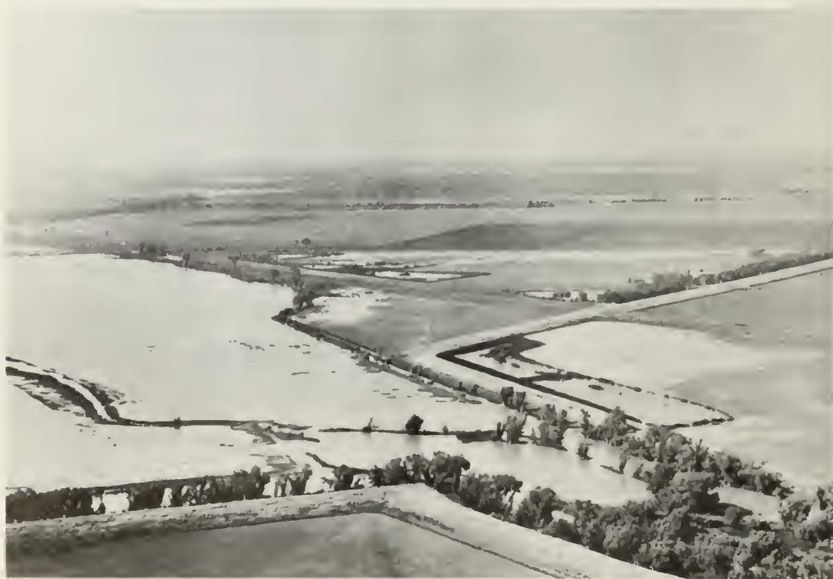
Any flow in excess of 100 second-feet crosses the Yolo Bypass as a sheet.
