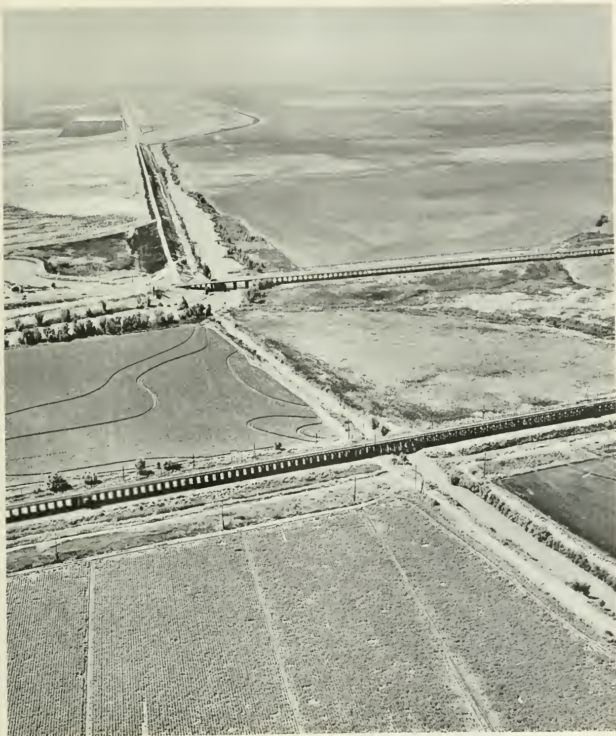
View of Tule Canal looking southward showing restricted channel capacity above Highway 40 crossing. Sacramento Deep Water Ship Channel and toe drain can be seen in background.
