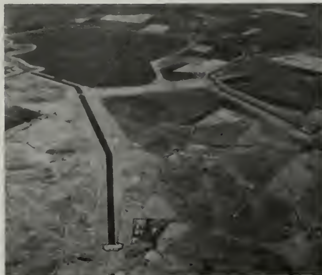
Clifton Court Forebay serves as the main Delta diversion point for the SWP. The Tracy Pumping Plant pumps water directly from Old River into the CVP Delta-Mendota Canal.
