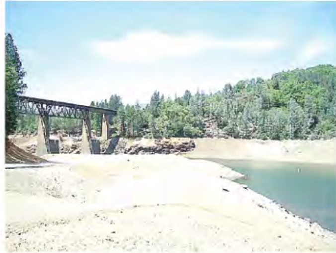
Sacramento Arm VAU, KOP 14, Photo 14b View looking northwest from Lower Salt Creek Road at the Salt Creek Resort.
