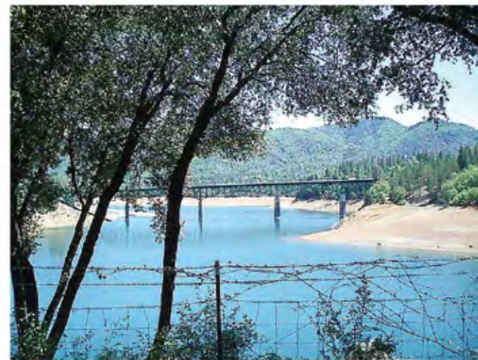
Sacramento Arm VAU, KOP 12, Photo 12a View looking east toward I-5 from the Lakeshore Resort Campground.
