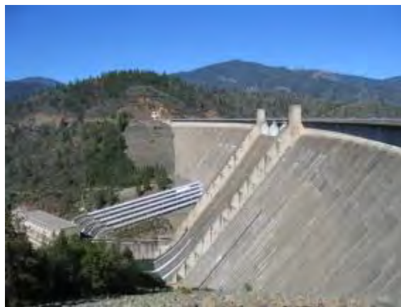
Figure 19-4. Shasta Dam and Infrastructure
