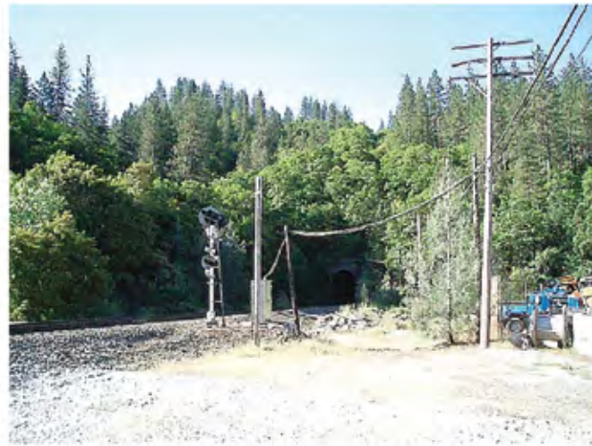
Bridge Bay VAU, KOP 3, Photo 3a View of the Union Pacific Railroad train tunnel looking south from the Bridge Bay Resort maintenance area.
