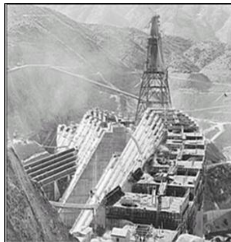
Shasta Dam Under Construction
