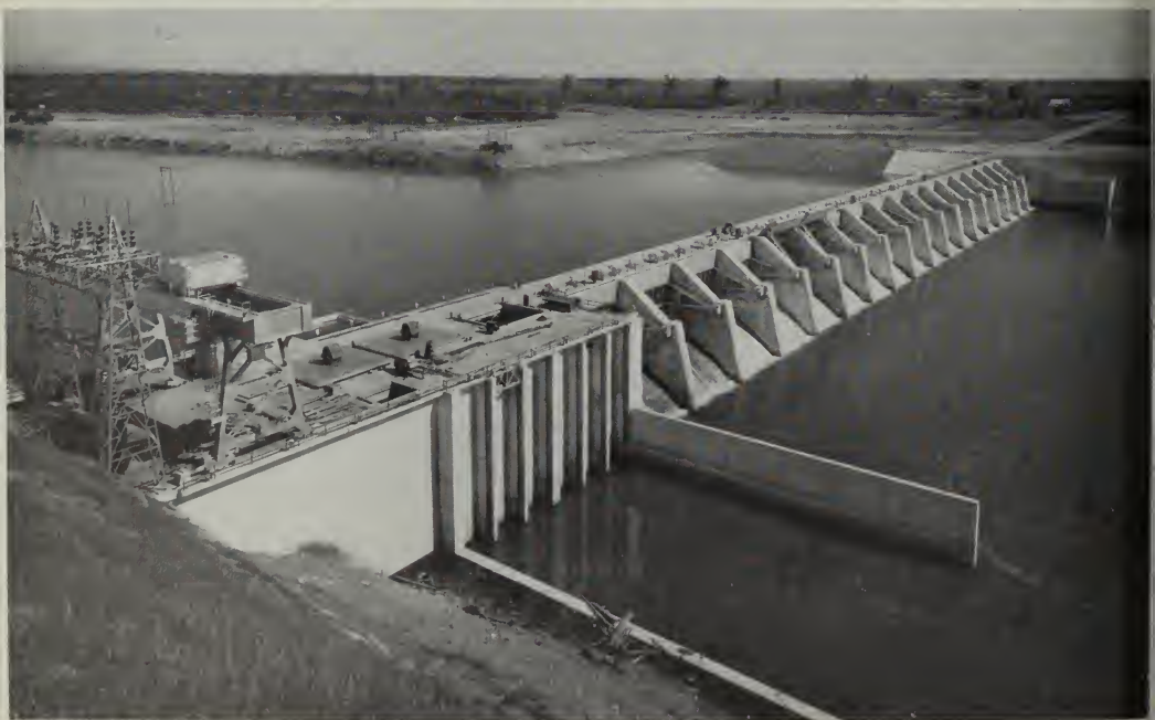
Sacramento Division—Constructed Features of the California Aqueduct System, Folsom and Nimbus Dams (top and bottom) on the American River
