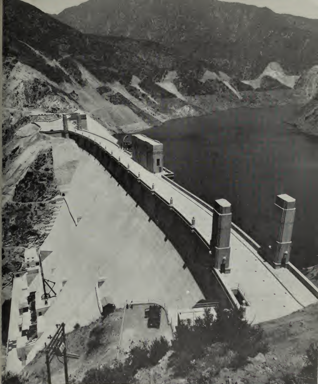
Southern California Division—The Proposed Terminal for the Chino-San Gabriel Aqueduct—Morris Reservoir Near Pasadena
