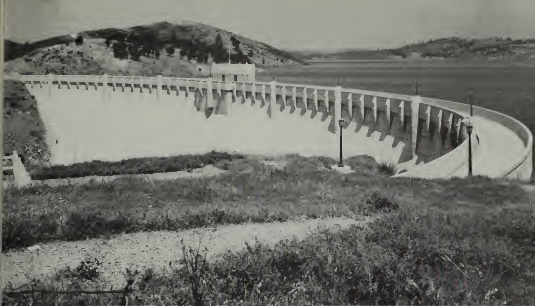
" . . . the East Bay area . . . has developed the waters of the Mokelumne River . . . " Pardee Dam
