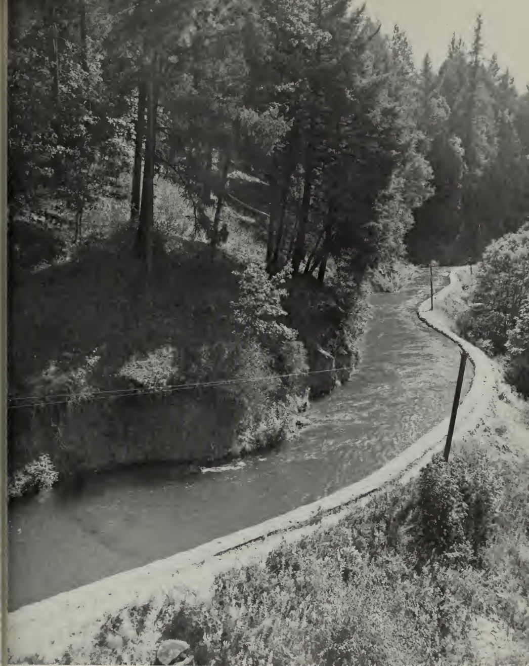
Sacramento River Basin—Bear River Canal in the Sierra Nevada, Constructed in 1850
