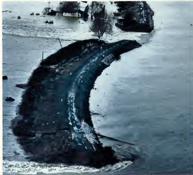
A levee on Tyler Island in the north Delta breaches during the 1986 floods. In all, six Delta islands and tracts flooded, as did Interstate 5 and numerous local roads. The flooding forced 1,600 people to evacuate and cost $20 million in direct damage.
