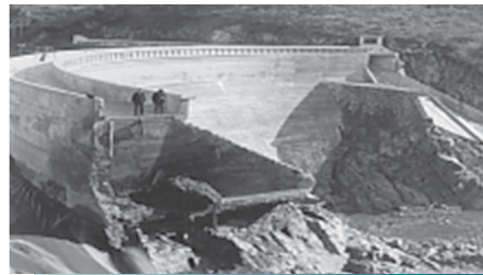
Example Sweetwater Dam Failure, 1916
