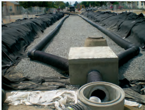
Photo A Elmer Avenue Infiltration Galleries Under Construction
