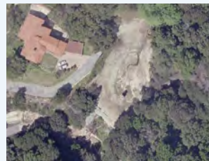
Photo B Mullally Debris Basin After Feb. 2010 Storms
