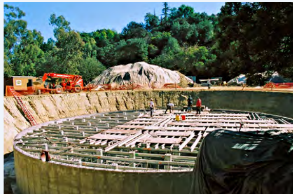
Photo A TreePeople’s 216,000-Gallon Cistern Under Construction
