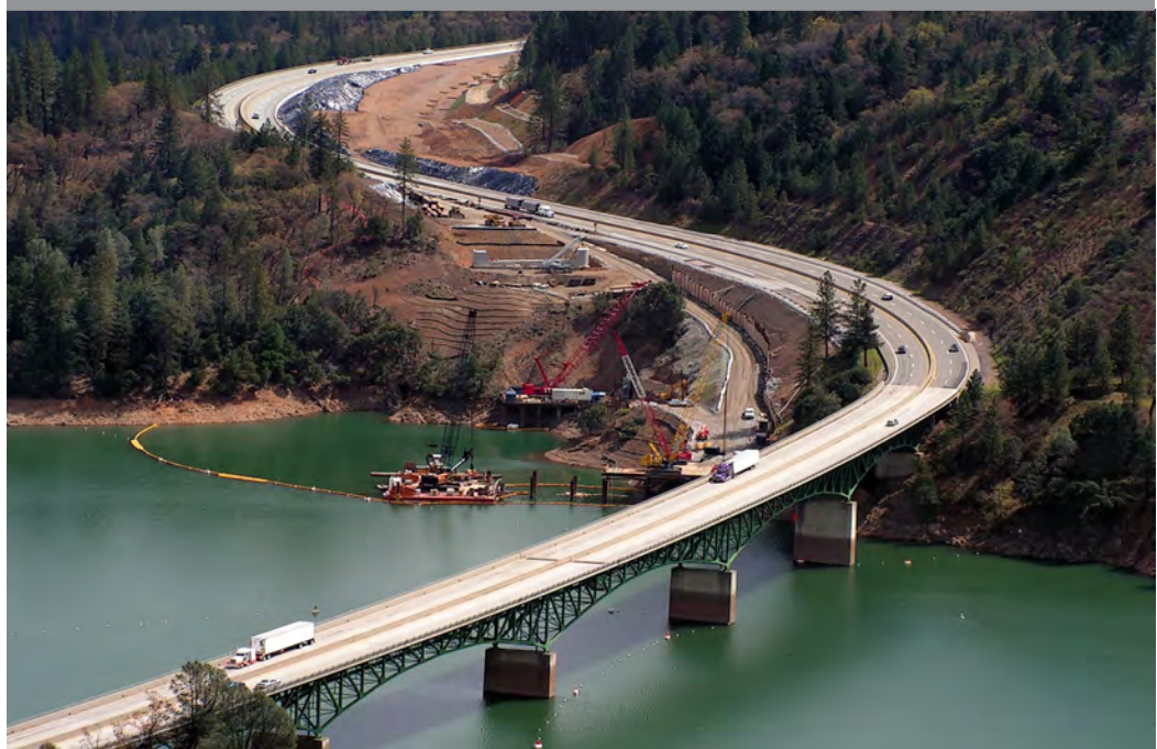
Photo 26-1 Caltrans I-5 Antlers Bridge Realignment Project on Shasta Lake
