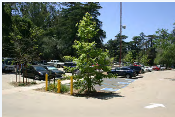
Photo B TreePeople’s Parking Lot with Storm Drains Piped to Cistern
