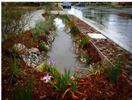
Photo B Elmer Avenue Curbside Bio-Swale Filled by Half-Inch Rainstorm
