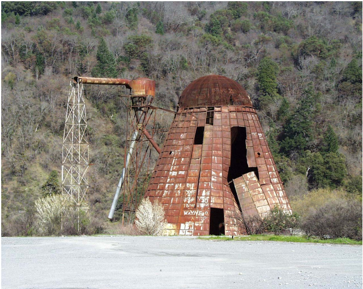
Tee-Pee Burner at Abandoned Cal-Pac Mill (2000)
