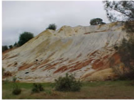
Improperly graded mine waste
