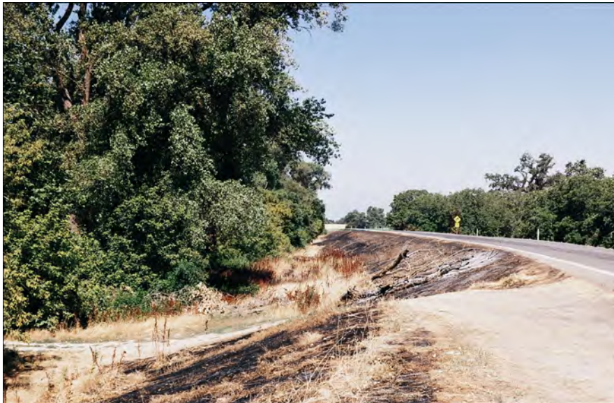
Figure 6-4. Riparian vegetation on waterside berm, downstream of Colusa Bridge
