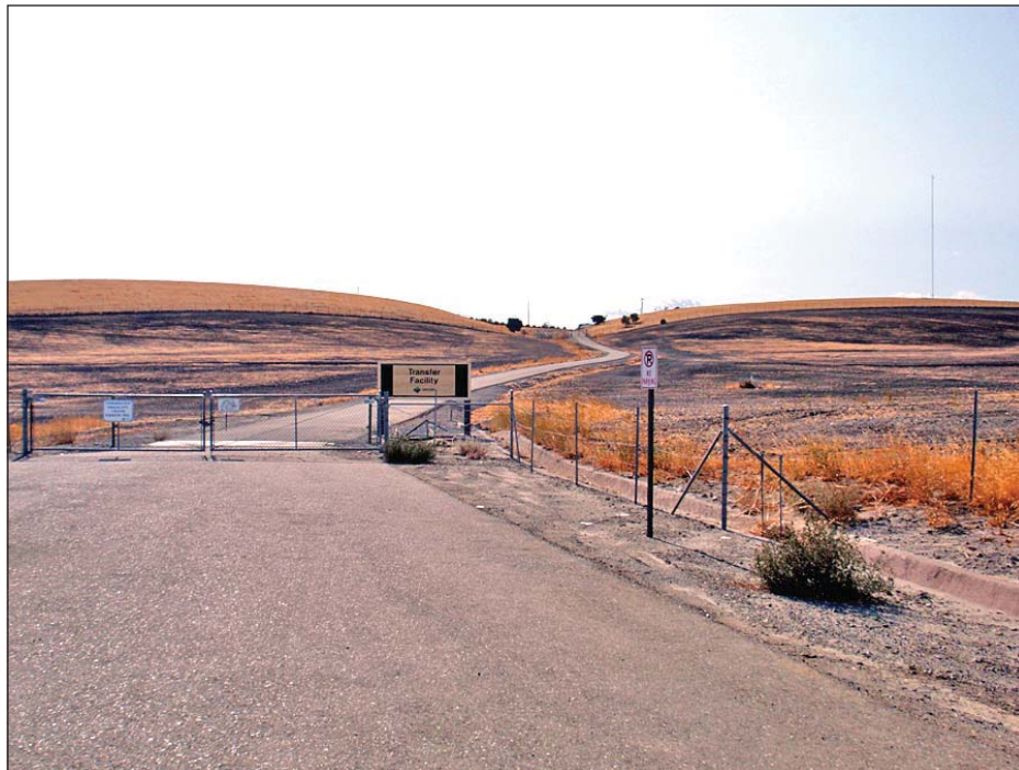
PHOTOGRAPH 10. View from Vasco Road looking southwest along Delta Transfer pipeline alignment to Transfer Facility (October 2008)
