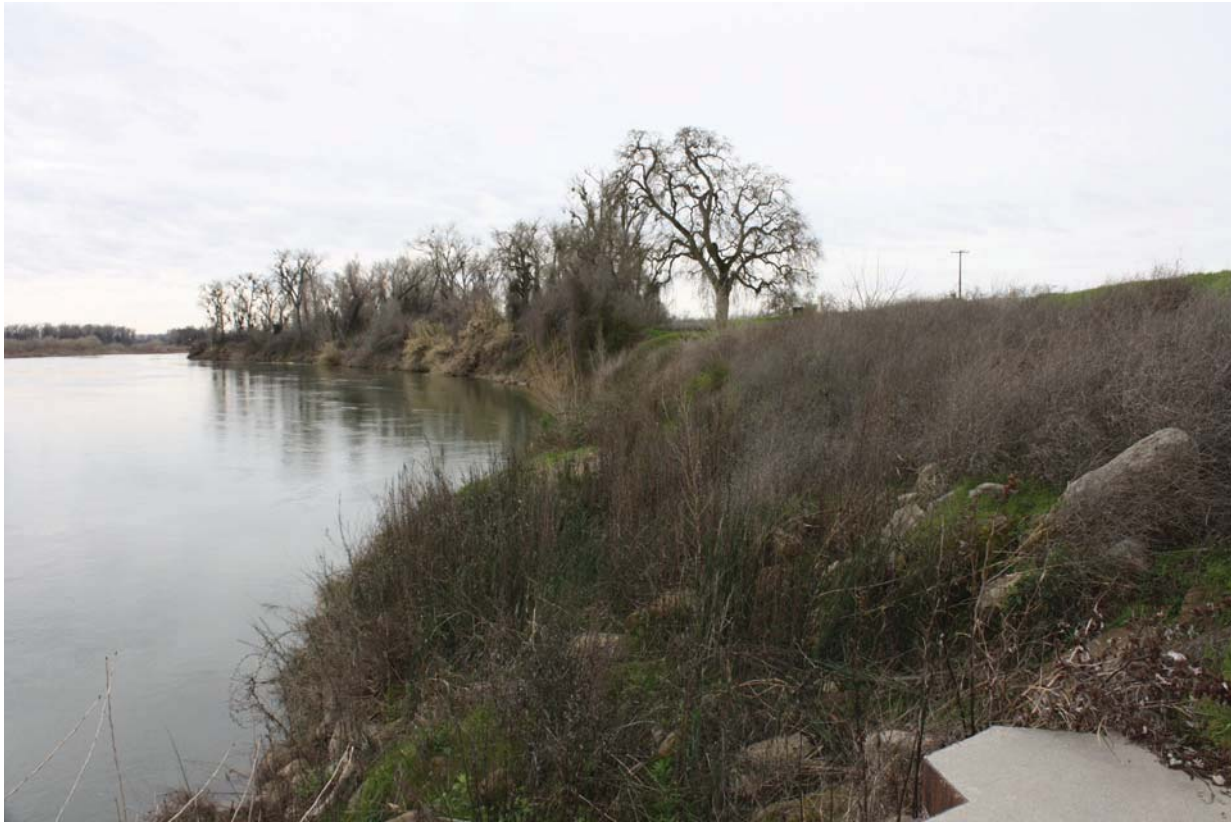
Photo 32: Looking south (downstream) from the Maxwell Irrigation District facility on the west side of the Sacramento River toward the Delevan Pipeline Intake and Discharge Facilities location.
