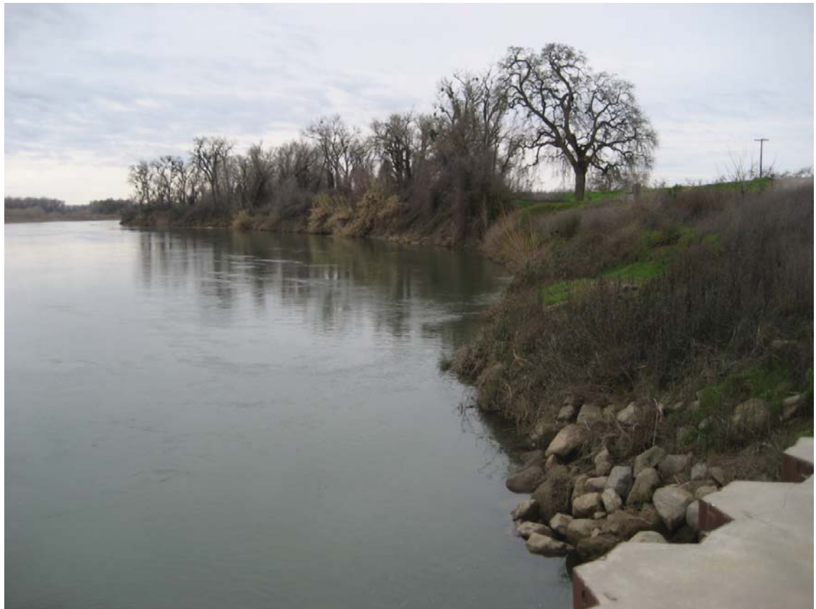
Location of the Proposed Delevan Pipeline Intake Facilities on the Sacramento River (Looking Downstream from the Existing Maxwell Irrigation District Intake) (2/23/2011)
