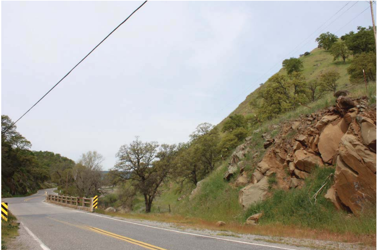
Photo 9: Looking west along Maxwell Sites Road toward the Sites Dam left abutment location, from outside of the inundation area.
