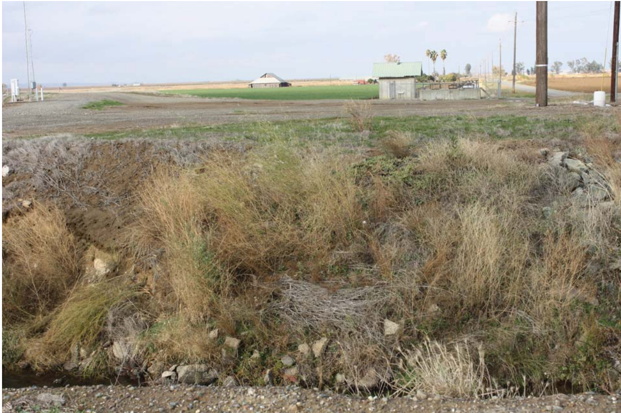
Photo 27: Looking northwest along the alignment of the TRR to Funks Creek Pipeline near the Outlet location at the Funks Creek crossing of McDermott Road.
