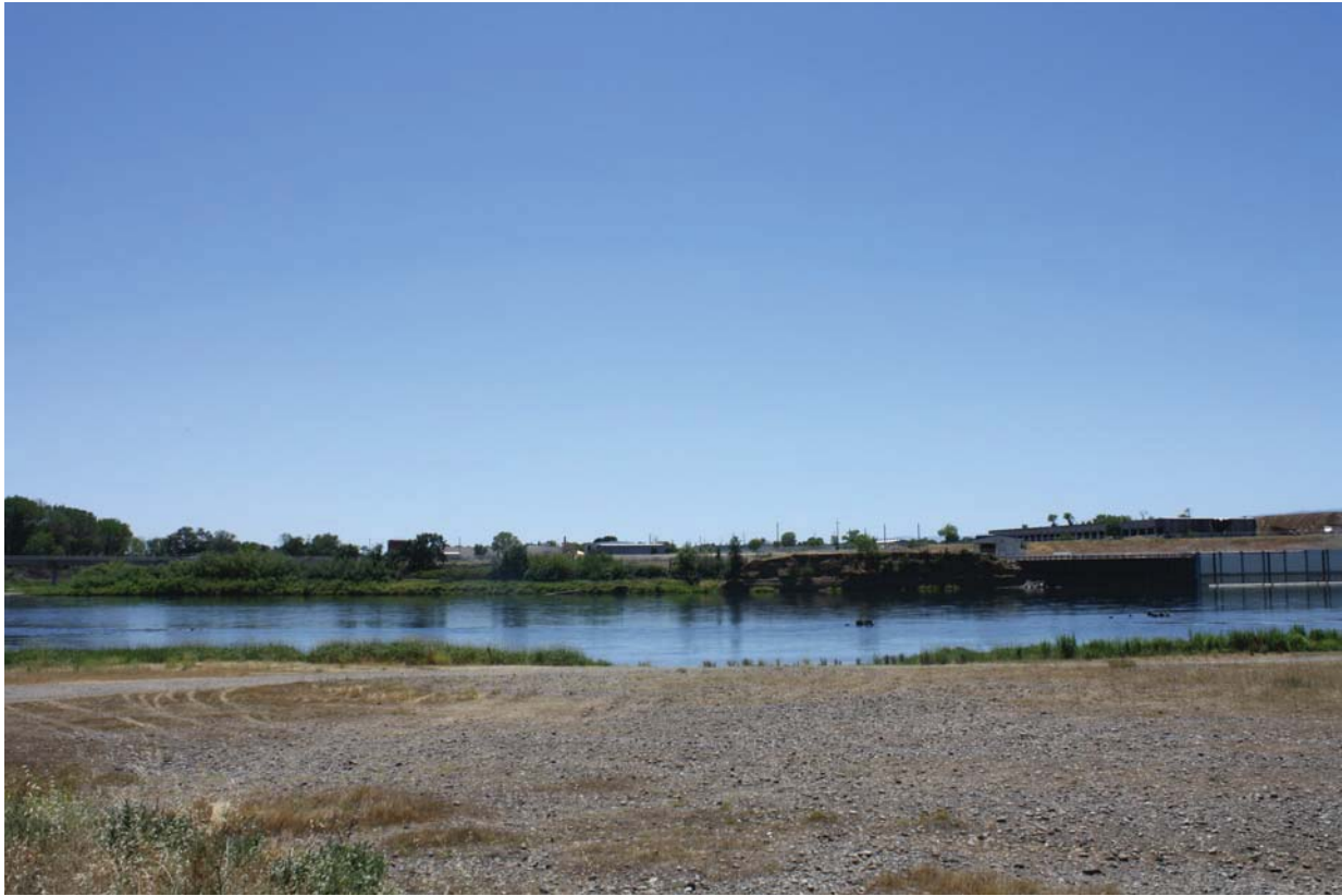
Photo 26: Looking west from the east side of the Sacramento River at the Red Bluff Pumping Plant.
