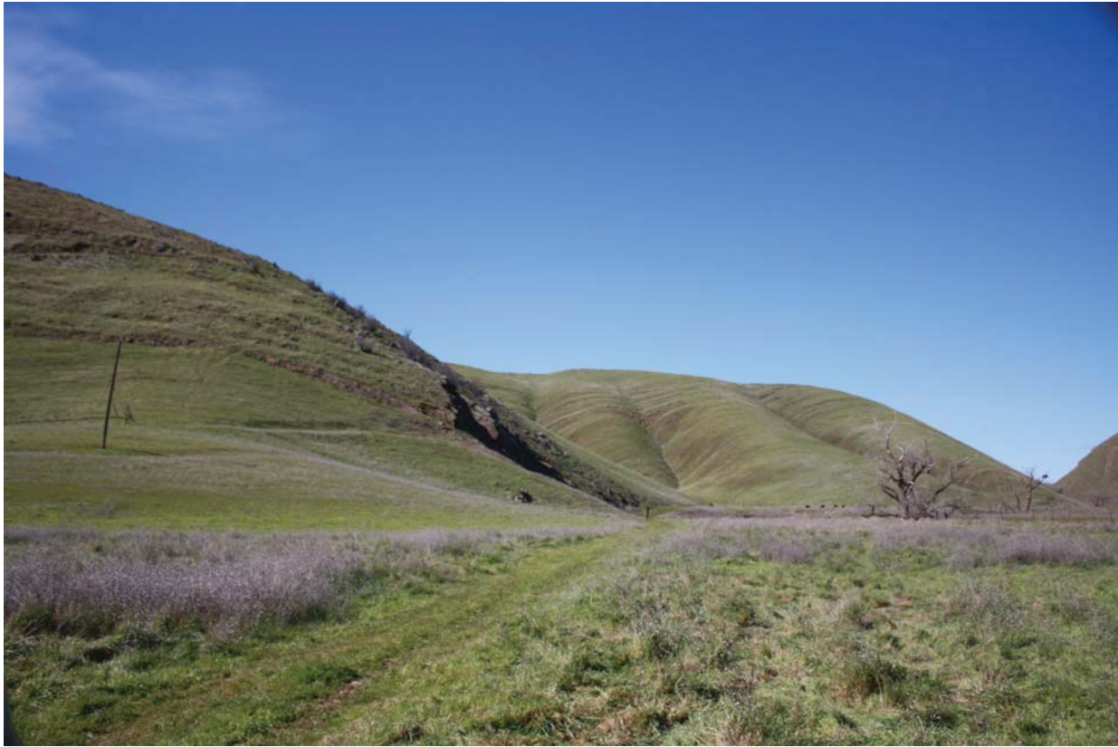
Photo 8: Looking northwest toward the Golden Gate Dam right abutment location from outside of the inundation area.
