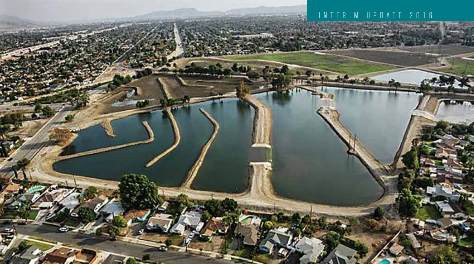
Pacoima spreading grounds (groundwater recharge facility) — San Fernando Valley
