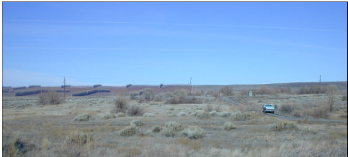
Photo 3.9-16. View of area near Vantage Substation
