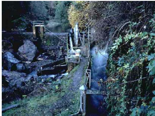
Eagle Canyon Diversion Dam
