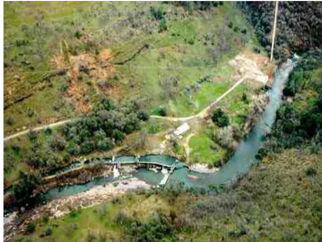
Coleman Diversion Dam and Inskip Powerhouse
