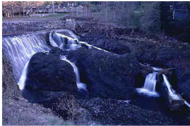
Inskip Diversion Dam
