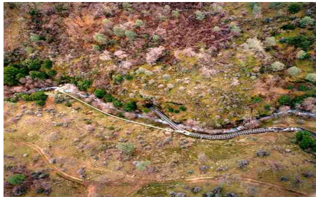
Soap Creek Feeder Diversion Dam
