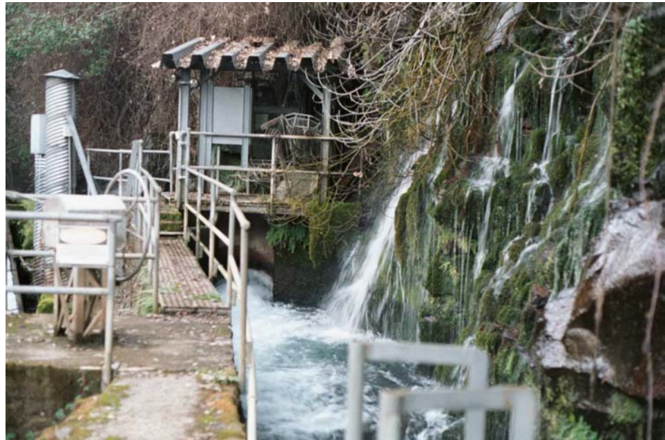
Figure 4.3-3 Spring Flow at Eagle Canyon Diversion Dam Flowing out of a Basalt Formation on the Southern Canyon Wall
