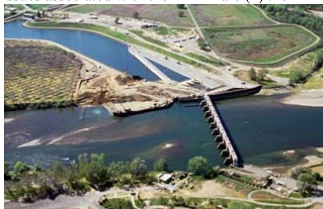
Red Bluff Diversion Dam on the Sacramento River
