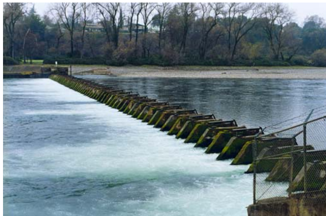
ACID Diversion Dam near Anderson Source: NOAA Photo Library
