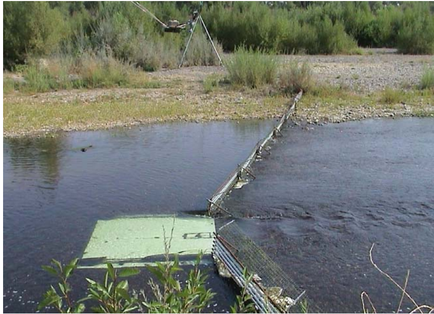
Figure 5. An example of a partial horizontal bar weir currently in use in the Upper Sacramento River Basin (Cottonwood Creek), operated to monitor fall-run Chinook salmon. The weir directs fish through the central opening where they are filmed by overhead and underwater cameras. Photo credit: Doug Killam, CDFG.
