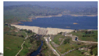
1949 Friant Dam was built
