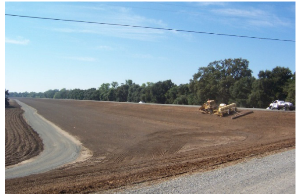
Construction of a new levee in the Natomas Basin of Sacramento
