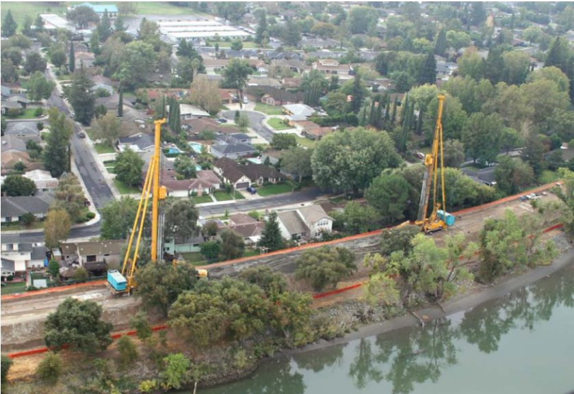
Geotechnical improvements to levees in the Pocket Area of Sacramento
