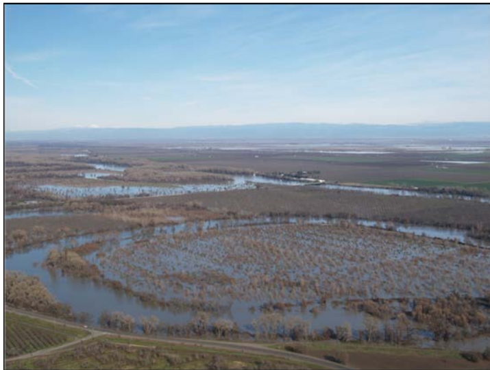
Setback levee at Butte City
