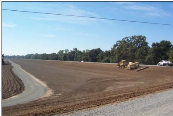
New levee construction at Natomas
