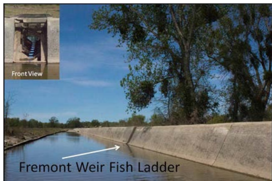
Fish Passage Constraints at Fremont Weir
