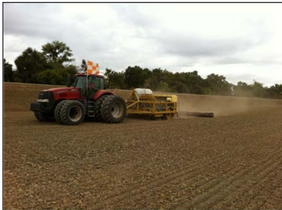
Planting native grass seeds on the Natomas levee
