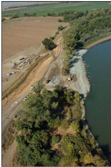
Levee repair on lower Sacramento River
