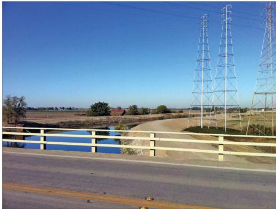
PHOTOGRAPH 1. Looking north from the Howard Road bridge crossing of the San Joaquin River. Vegetation along the river is mostly absent, while the vegetation data identifies the left bank as Himalayan blackberry stands and the right bank as riparian scrub. This inaccuracy may be a result of periodic maintenance that removes vegetation or incorrect habitat mapping.
