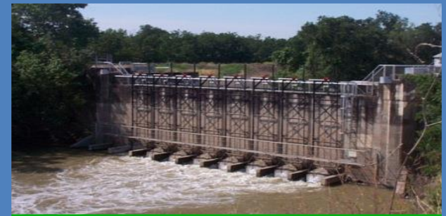
Knight's Landing Outfall Gates
