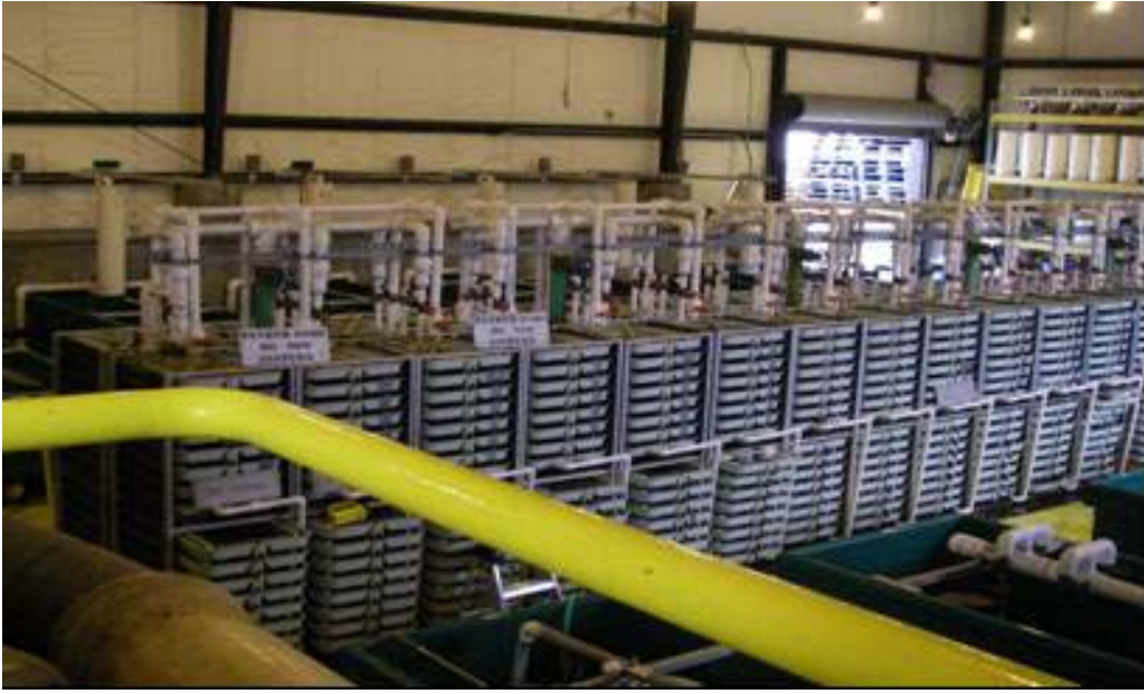
Figure 4-16. Vertical 16-tray egg incubators in NFH Building 2.
