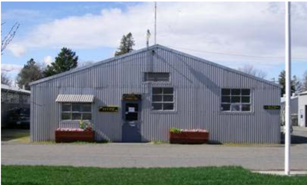
Figure 4-25. Exterior of the Fish NFH Headquarters/Office Building.
