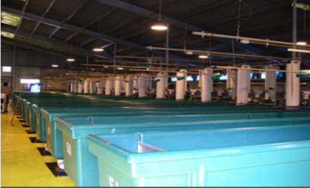
Figure 4-18. Interior of NFH Building 1.
