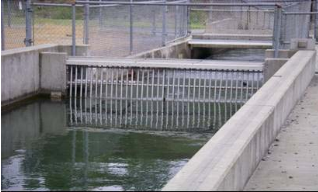
Figure 4-6. Fish trap at the top of the fish ladder facing north.
