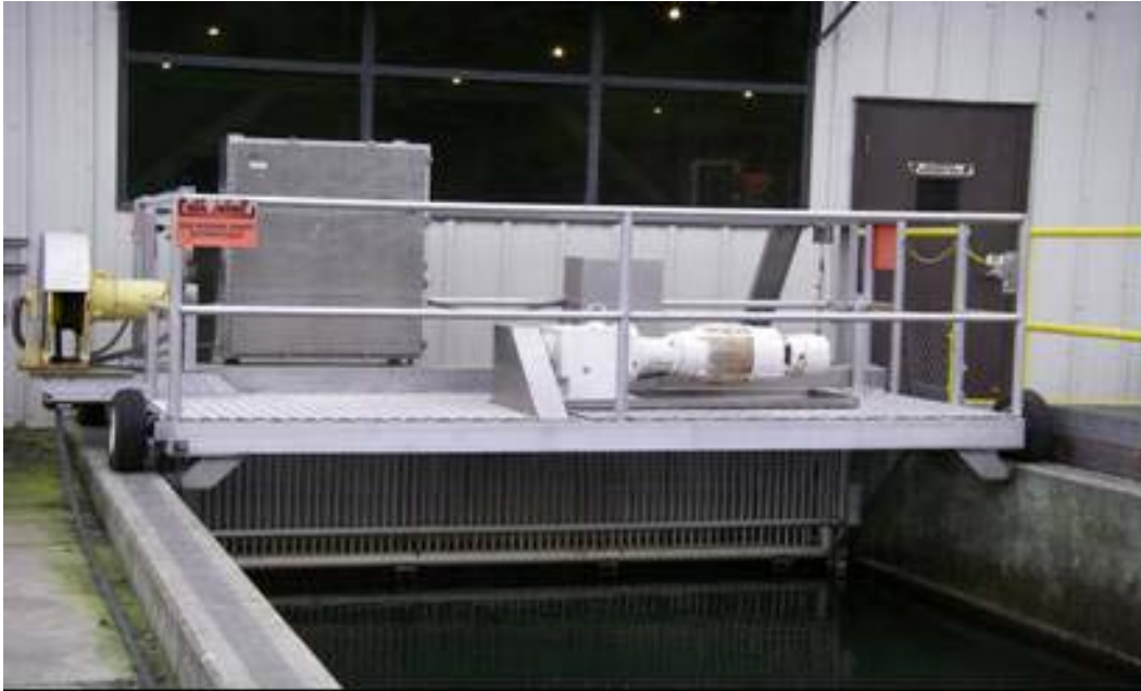
Figure 4-7. Electric/hydraulic fish crowder in the adult holding pond.
