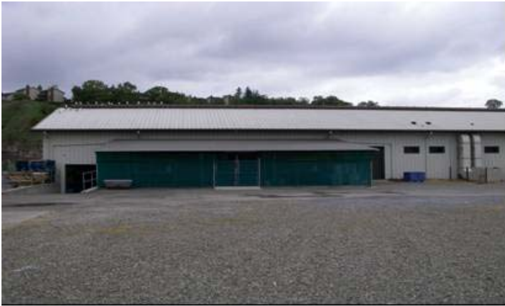
Figure 4-12. Exterior of NFH Building 2.
