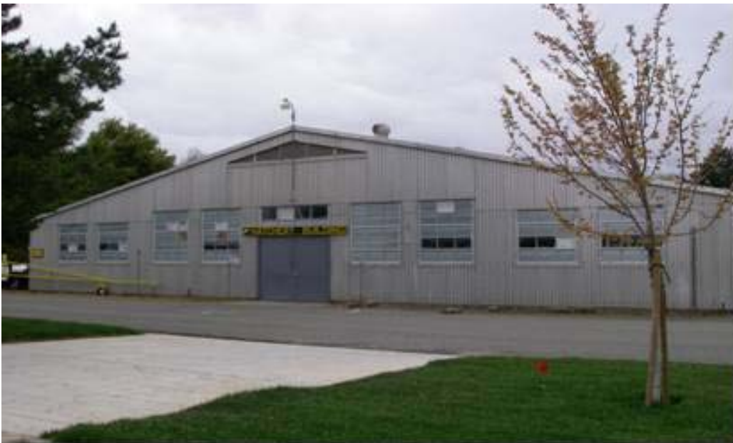
Figure 4-17. Exterior of NFH Building 1.
