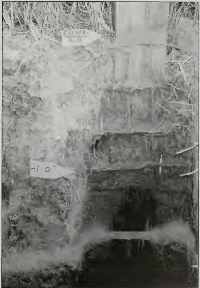
Figure 5. Exposure showing accretion of 1.3 ft of sediments on "upstream" side of Highway 101 at T-4 (Figures 1 and 4), and the now-buried five lower wires of the 10-strand mesh. The 1954 ground surface is shown by the light-colored line in the lower part of the photograph.
