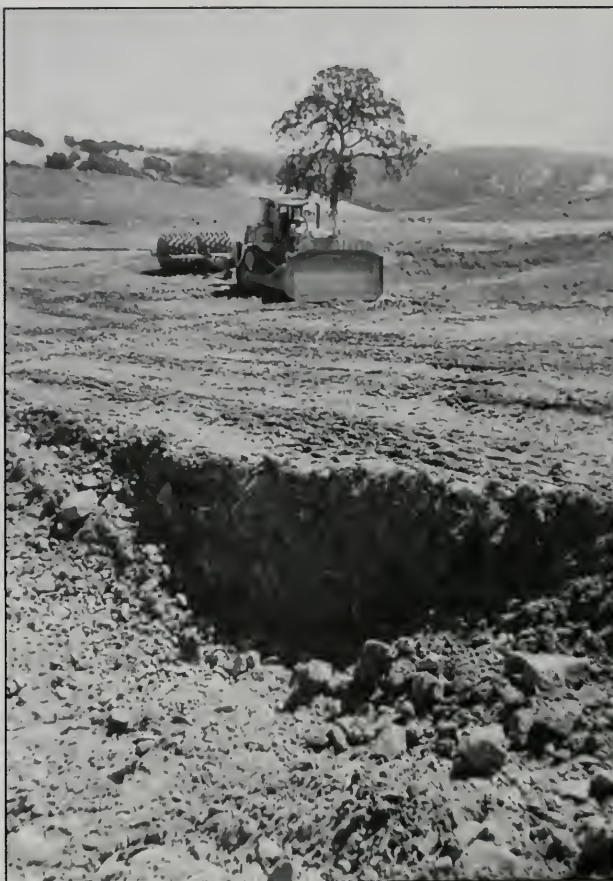
Figure 4. Dozer pit excavated for visual observation.
