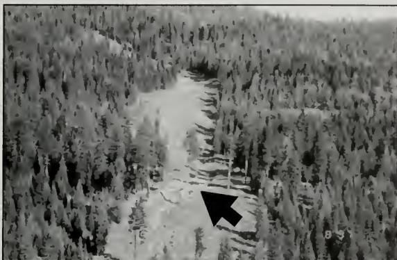
Figure 6. The upper part of the debris flow runout. California Highway 4 crosses the runout in the middle of this photo, where a Caltrans dump truck is visible (arrow).
