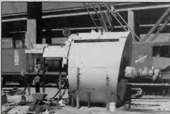
Figure 18. Tunnel shield with roadheader excavator.
