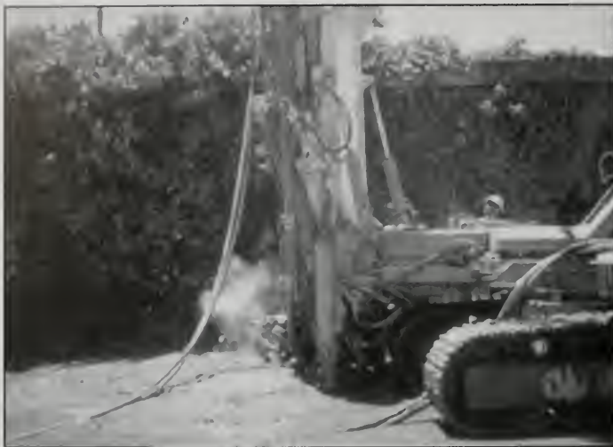
Figure 12. Installing jet grouted columns for tunnels.
