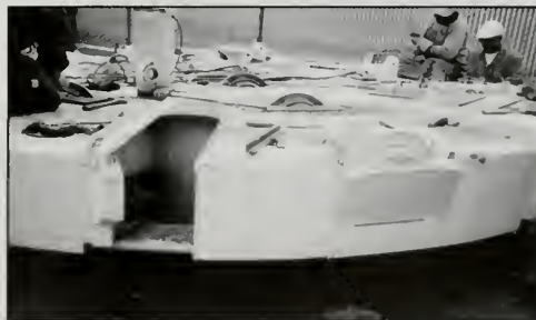
Figure 3. Fabricating TBM cutterhead on-site.
