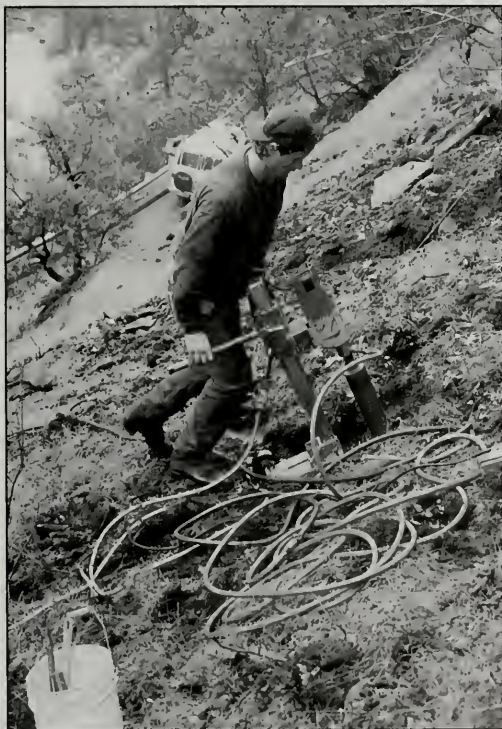
Figure 3. Contractor drilling for net anchor. Note the steep, loose terrain.
