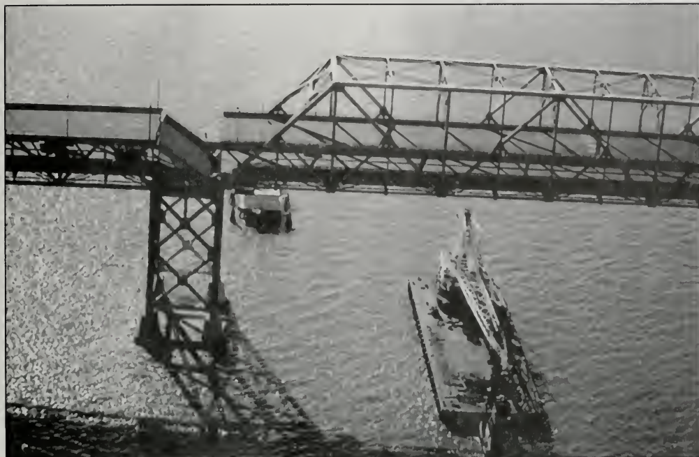
Figure 2. Photograph of damage to the east span of the bridge from the 1989 Loma Prieta earthquake.
