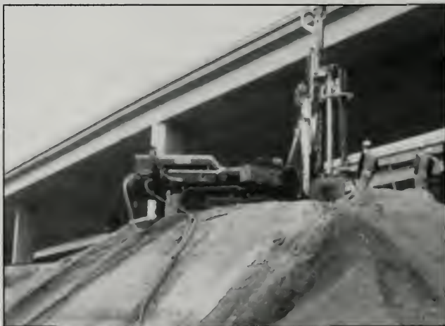
Figure 17. Jet grouting under the commuter railroad embankment.
