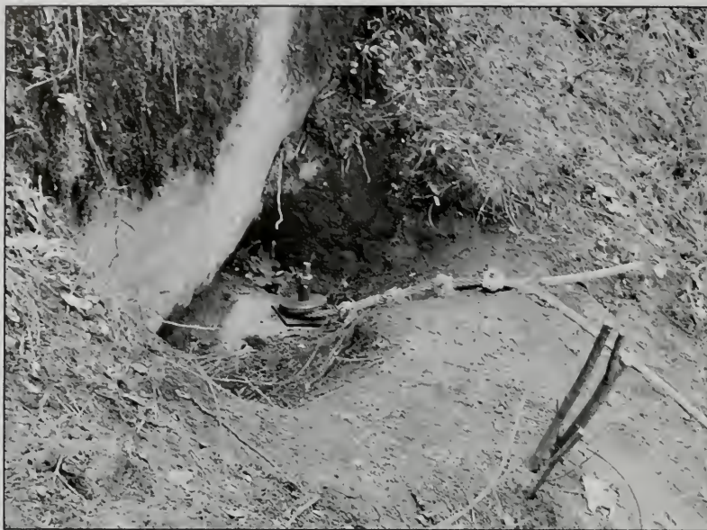
Figure 5. Finished cable net anchor grouted in place with cable attached.
