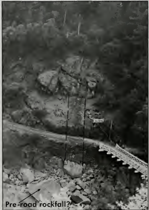
Figure 2. View south across American River after rockfall. Note the skid path left of the bridge, and the large angular boulder in the bottom left.
