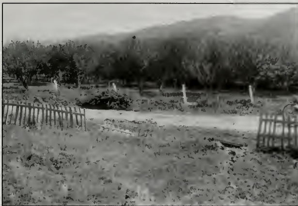
Figure 8. En echelon cracks of the Woodside trace crossing Portola Road in 1906. View to the south. Stanford University Archives, J.C. Branner collection. Courtesy of the U.S. Geological Survey.
