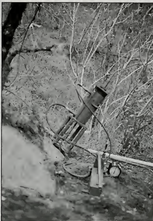
Figure 4. Testing anchor pull-out resistance capacity, using a Williams Form 60-ton jack.
