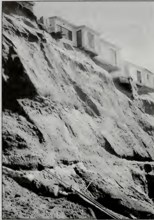
Figure 1. Residences along Esplanade Avenue, Pacifica, in danger of collapse in February, 1998.
