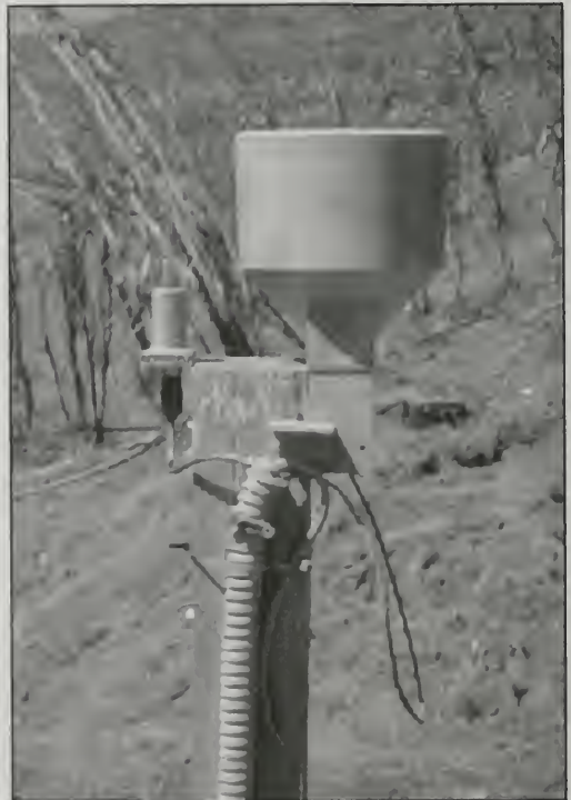
Figure 8. Total station system allowing remote website monitoring of slope inclinometers, piezometers, and downhole extensometers.
