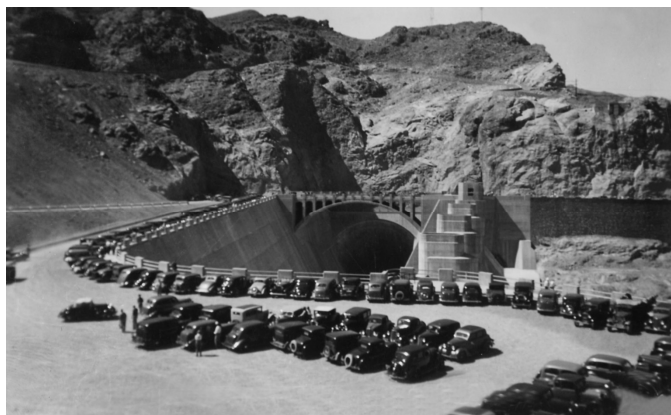
FIG. 17. Once the dam was dedicated and opened to the public the National Park Service had to cope with traffic congestion and finding suitable parking areas. This 1938 view shows the first parking lot, just upstream of the voluminous Arizona Spillway intake. Another higher lot, from which this photo was taken, was added a short while later. Visitors walked to the dam and took the public elevator down to the power house (USBR).
