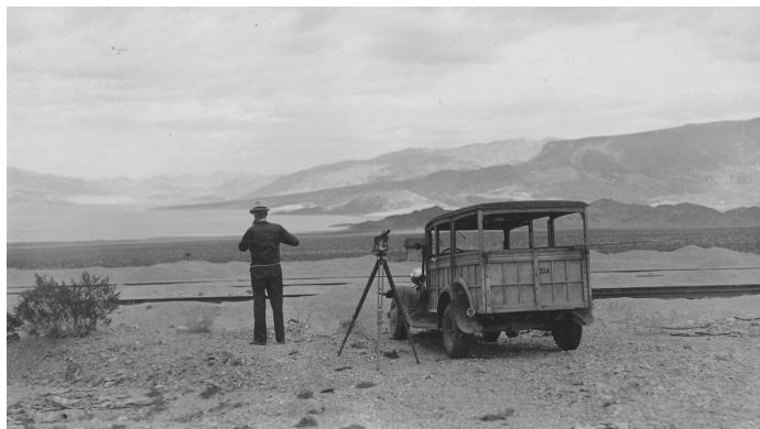
FIG. 1. Triangulation surveying of established monuments around Lake Mead began in 1935, to ascertain the extent of crustal deformation caused by the weight of the rising reservoir (USBR).
