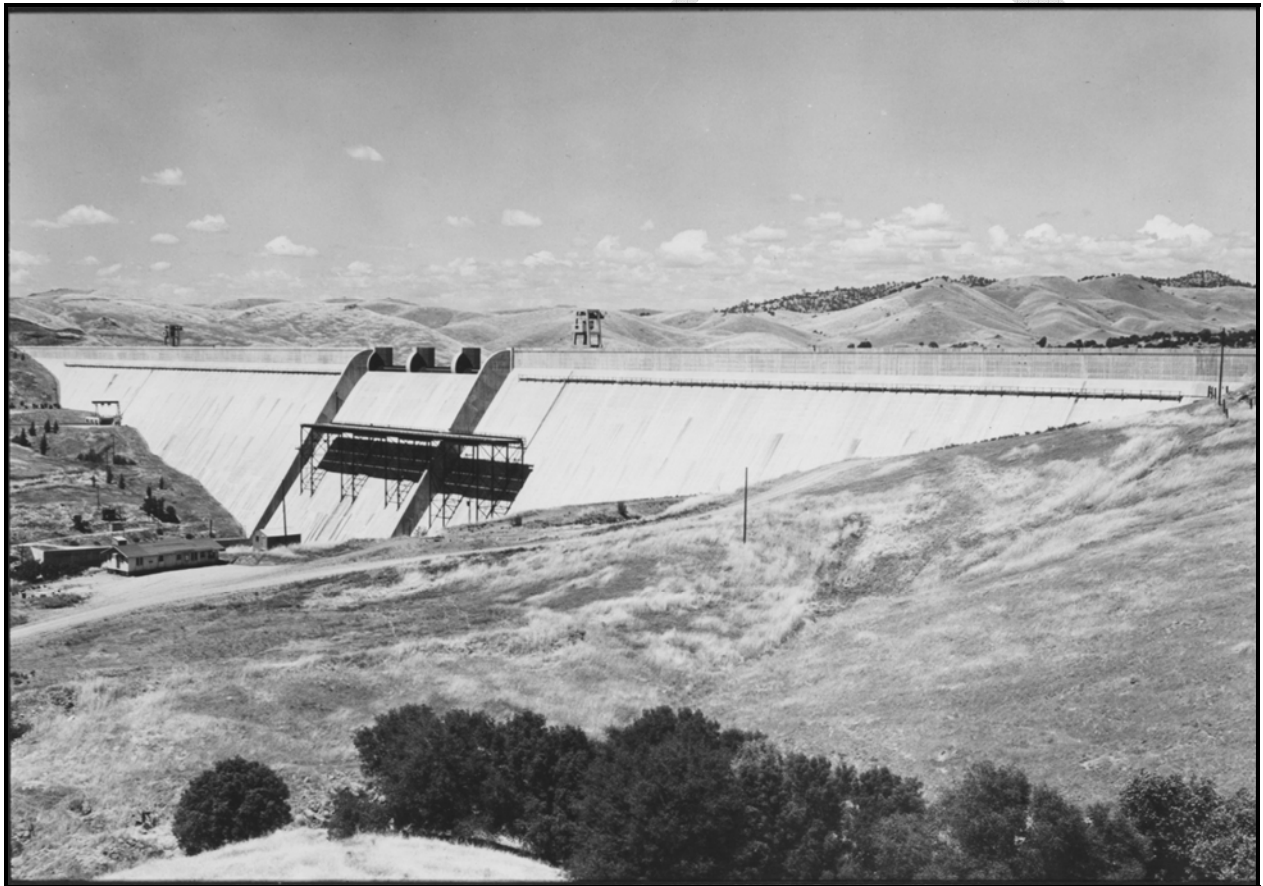
Friant Dam Nearing Completion, 1942 (Bureau of Reclamation)
