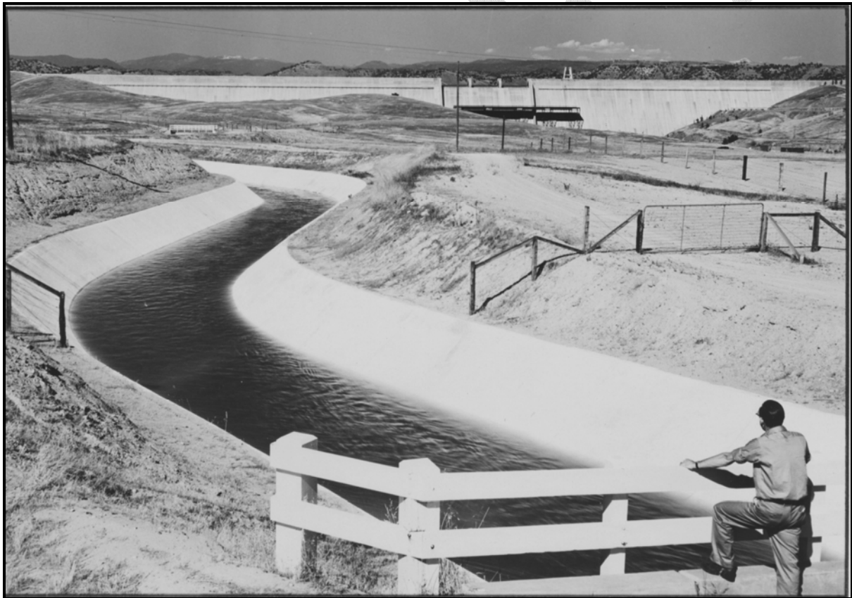
Madera Canal, With Friant Dam in Background (Bureau of Reclamation)
