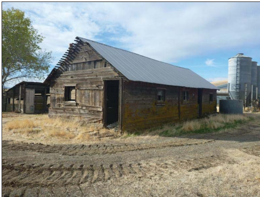
Figure 11: Edward Owens Farmstead, Bunkhouse, view looking southwest (C. Jimenez, November 13, 2012).
