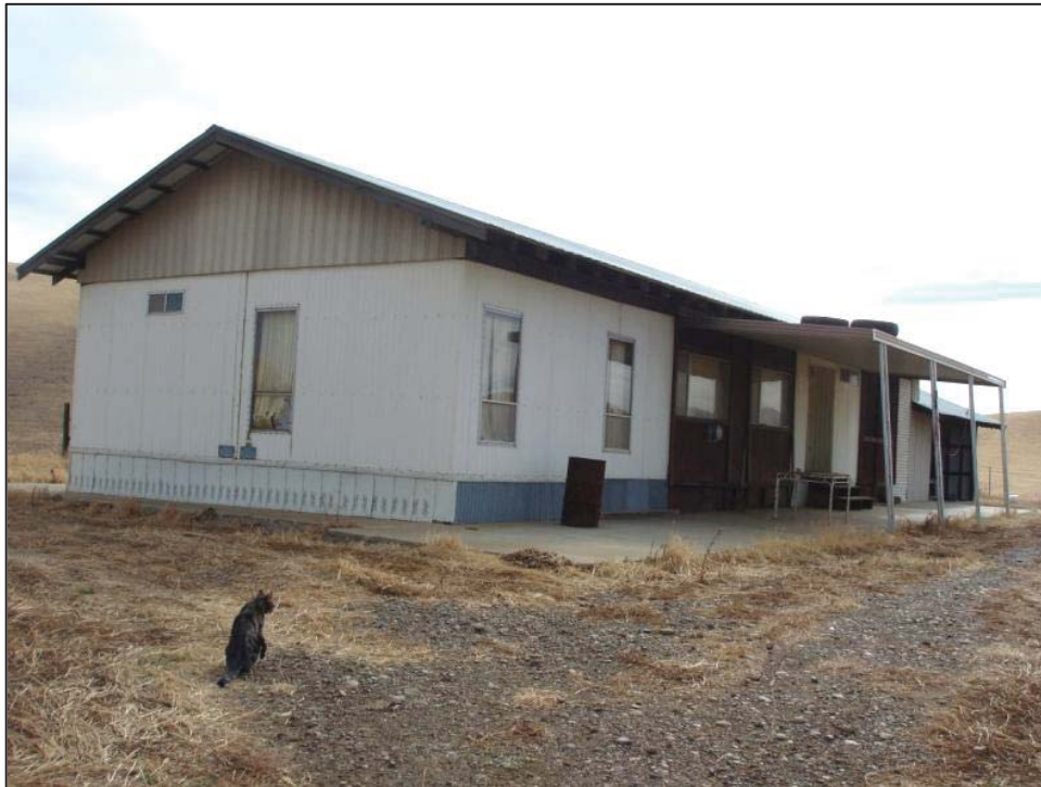
Figure 39: Edward Owens Farmstead, Double-wide mobile home, view looking southeast (C. Jimenez, November 13, 2012).
