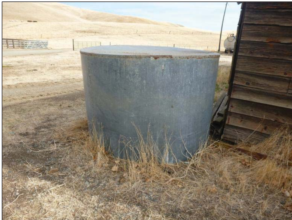
Figure 14: Edward Owens Farmstead, Water tank, view looking northeast (C. Jimenez, November 13, 2012).
