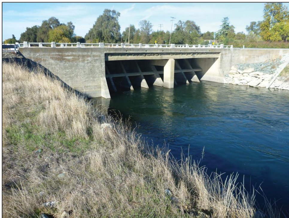
Figure 10: GCID Headgate, south elevation (C. Jimenez, November 14, 2012).
