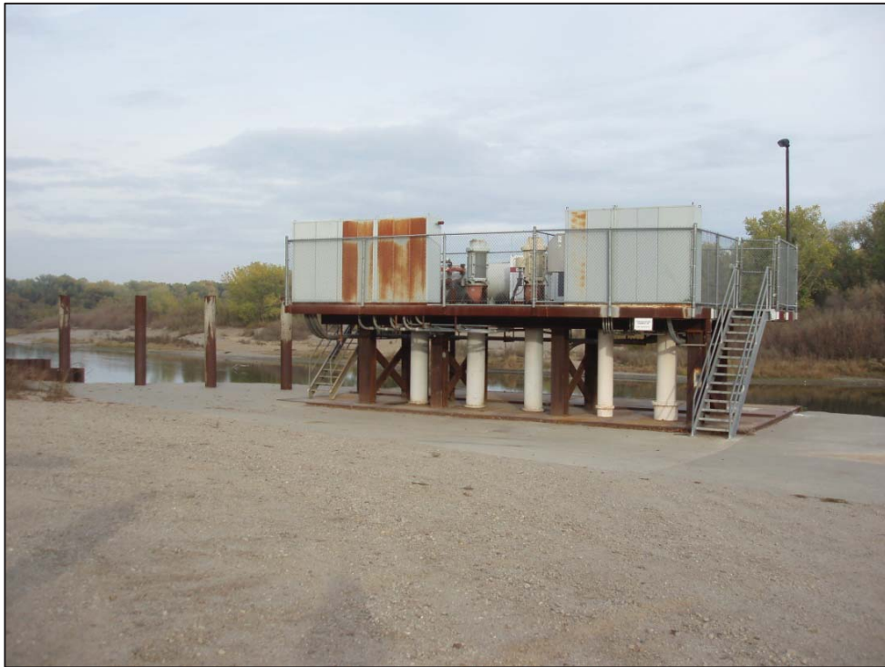
Figure 1: Maxwell Irrigation District, New pumphouse, view looking northeast (C. Jimenez, November 13, 2012).
