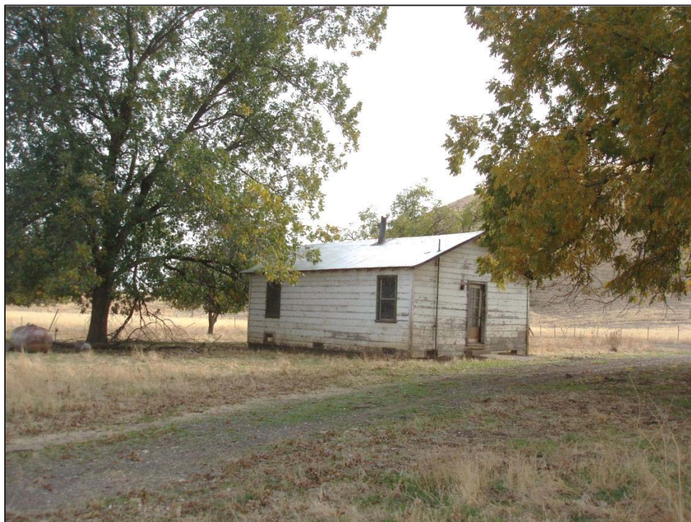
Figure 1: Shirley Jensen Farmstead, House, view looking southeast (C. Jimenez, November 13, 2012).
