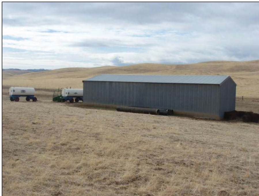
Figure 45: Edward Owens Farmstead, Bank barn 2, view looking east (C. Jimenez, November 13, 2012).
