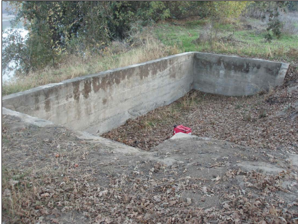
Figure 3: Maxwell Irrigation District, Concrete foundation, view looking southeast (C. Jimenez, November 13, 2012).
