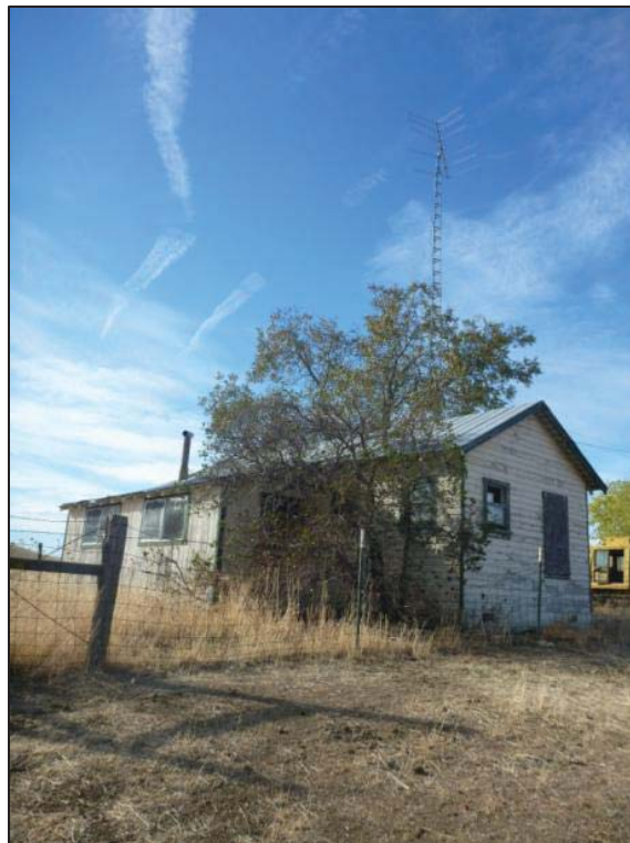
Figure 2: Edward Owens Farmstead, House, view looking southwest (C. Jimenez, November 13, 2012).
