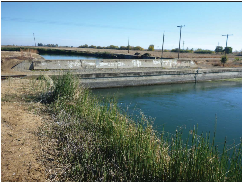
Figure 2: Union Pacific Railroad siphon, view looking northeast (C. Jimenez, November 14, 2012).
