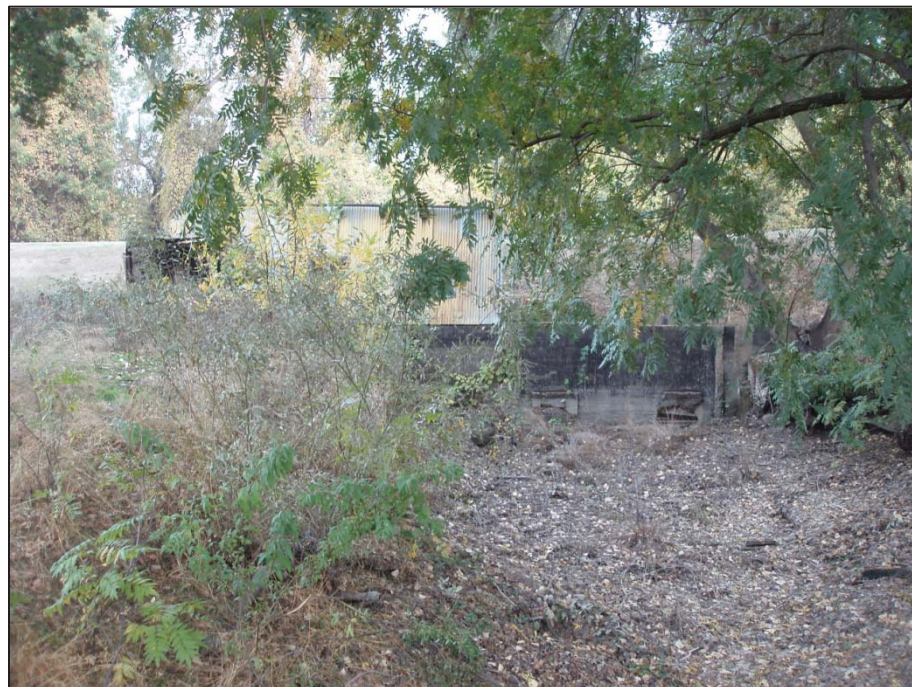
Figure 16: Maxwell Irrigation District, Abandoned pumpstation, view looking east (C. Jimenez, November 13, 2012).
