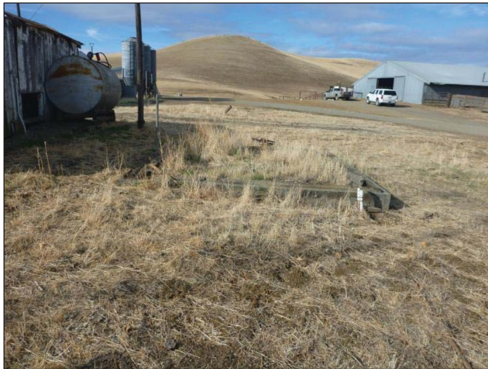
Figure 8: Edward Owens Farmstead, concrete foundation, view looking west (C. Jimenez, November 13, 2012).
