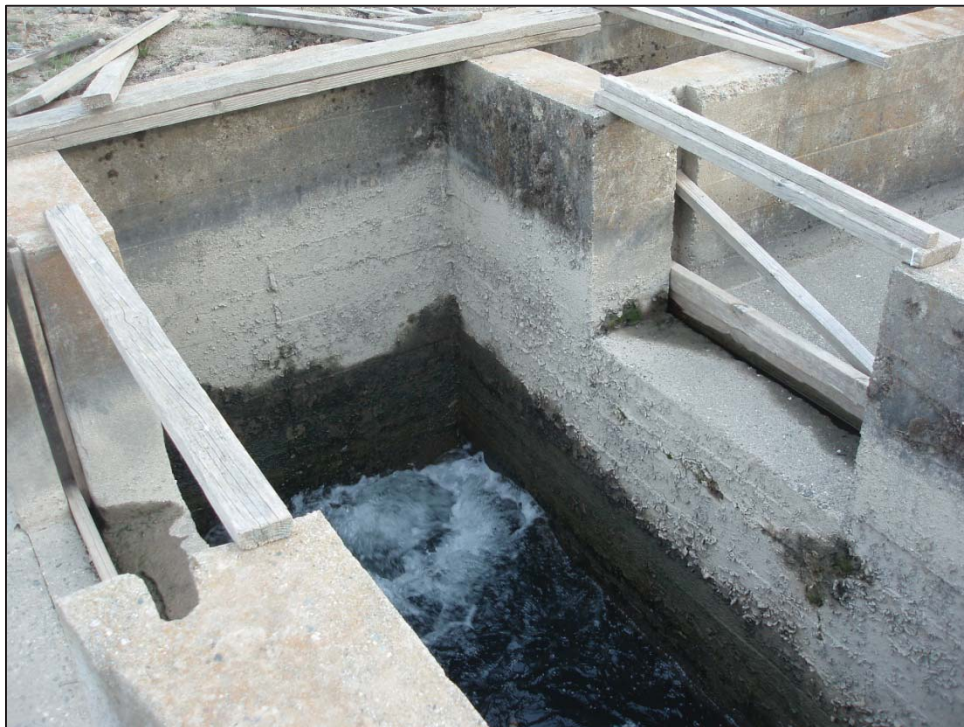
Figure 10: Maxwell Irrigation District, Concrete irrigation box culvert, detail (C. Jimenez, November 13, 2012).
