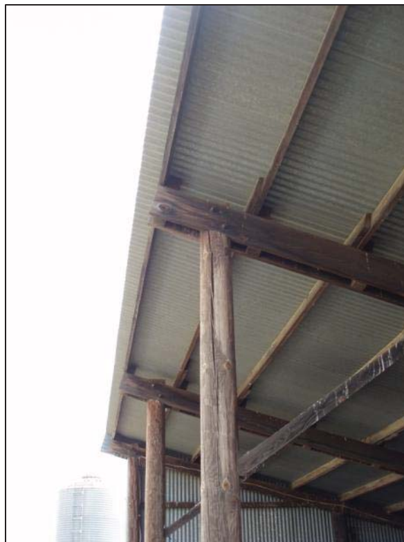
Figure 28: Edward Owens Farmstead, Bank barn 1, roof detail (C. Jimenez, November 13, 2012).
