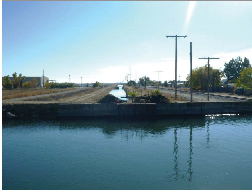
Figure 5: Union Pacific Railroad siphon from Glenn Colusa Irrigation Canal down an intersecting conveyance feature, view looking south (C. Jimenez, November 14, 2012).
