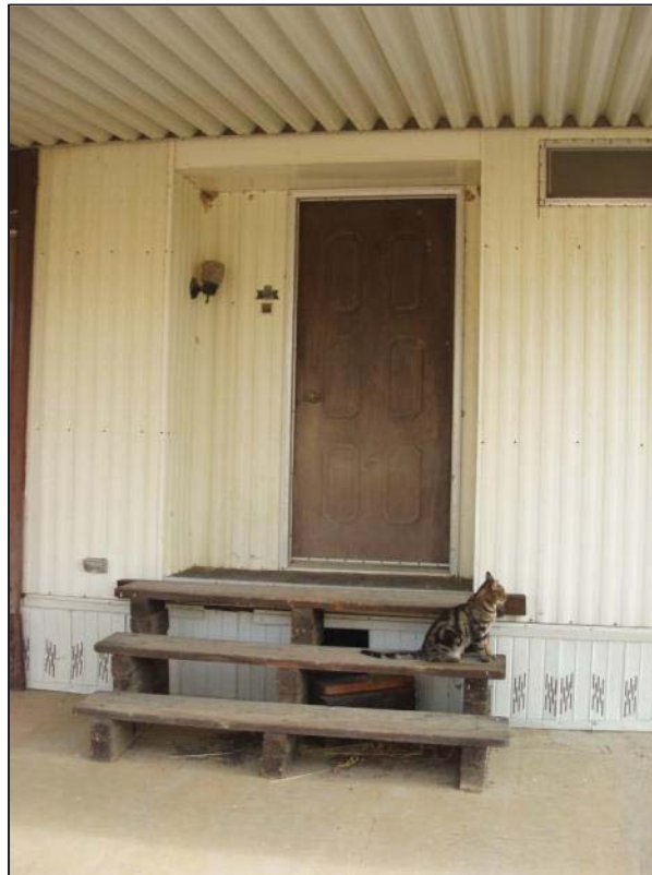
Figure 43: Edward Owens Farmstead, Double-wide mobile home, entrance, view looking east (C. Jimenez, November 13, 2012).
