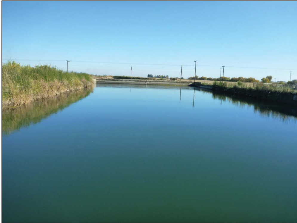
Figure 1: Union Pacific Railroad siphon, view looking east (C. Jimenez, November 14, 2012).
