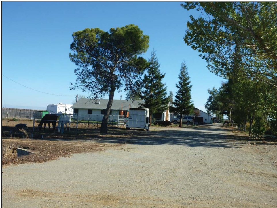
Figure 6: 4790-92 McDermott Road, House and outbuildings, view looking east (C. Jimenez, November 14, 2012).
