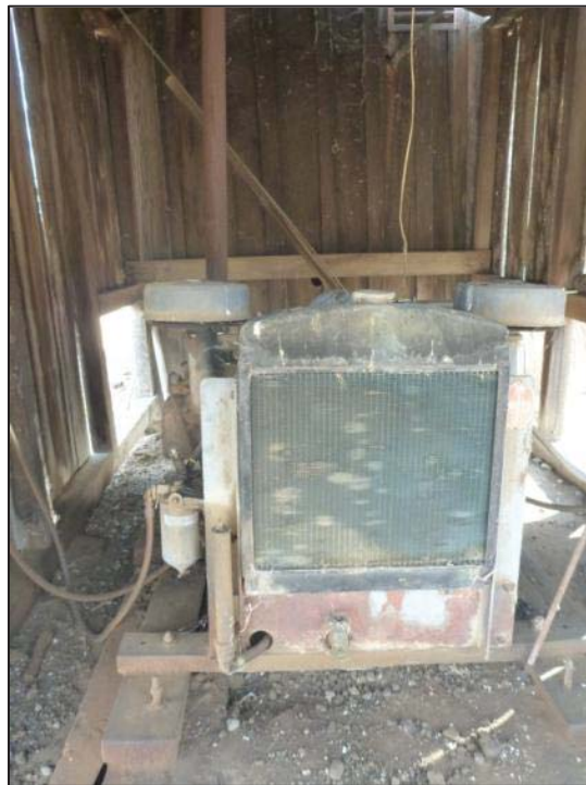
Figure 9: Edward Owens Farmstead, Shed A, interior detail . Note, old car engine as generator C. Jimenez, November 13, 2012).
