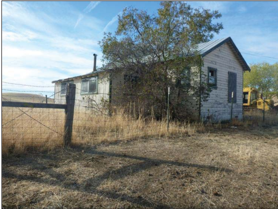
Figure 1: Edward Owens Farmstead, House, view looking southwest (C. Jimenez, November 13, 2012).
