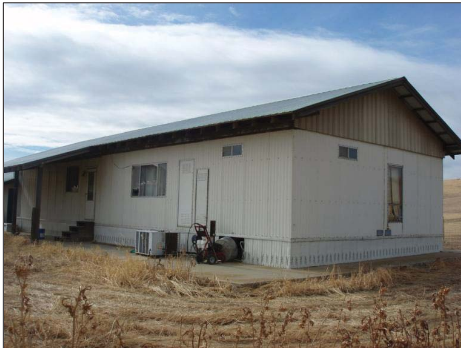
Figure 40: Edward Owens Farmstead, Double-wide mobile home, view looking southwest (C. Jimenez, November 13, 2012).
