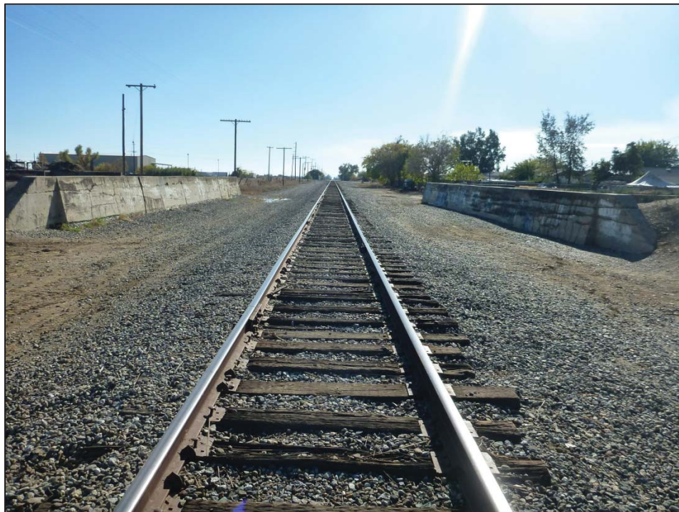
Figure 4: Union Pacific Railroad siphon from the railroad bed, view looking south (C. Jimenez, November 14, 2012).
