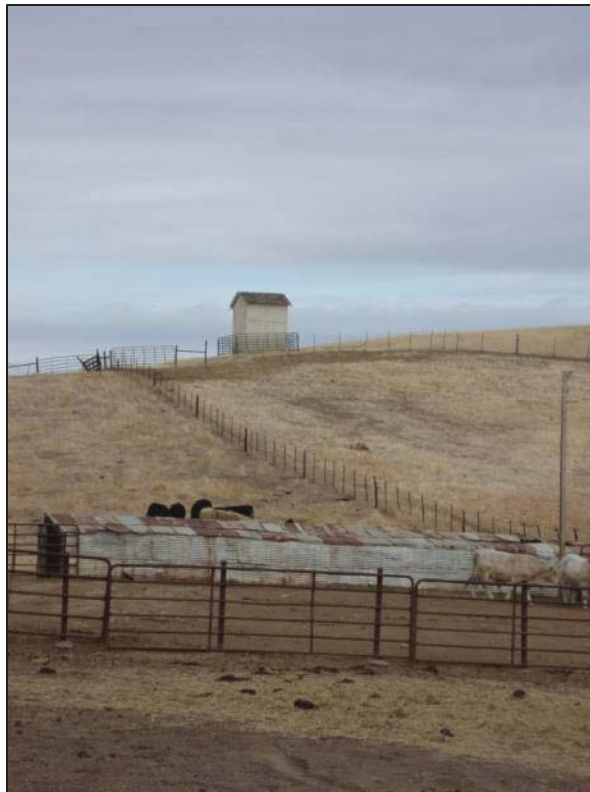
Figure 46: Edward Owens Farmstead, Pumphouse, view looking north (C. Jimenez, November 13, 2012).
