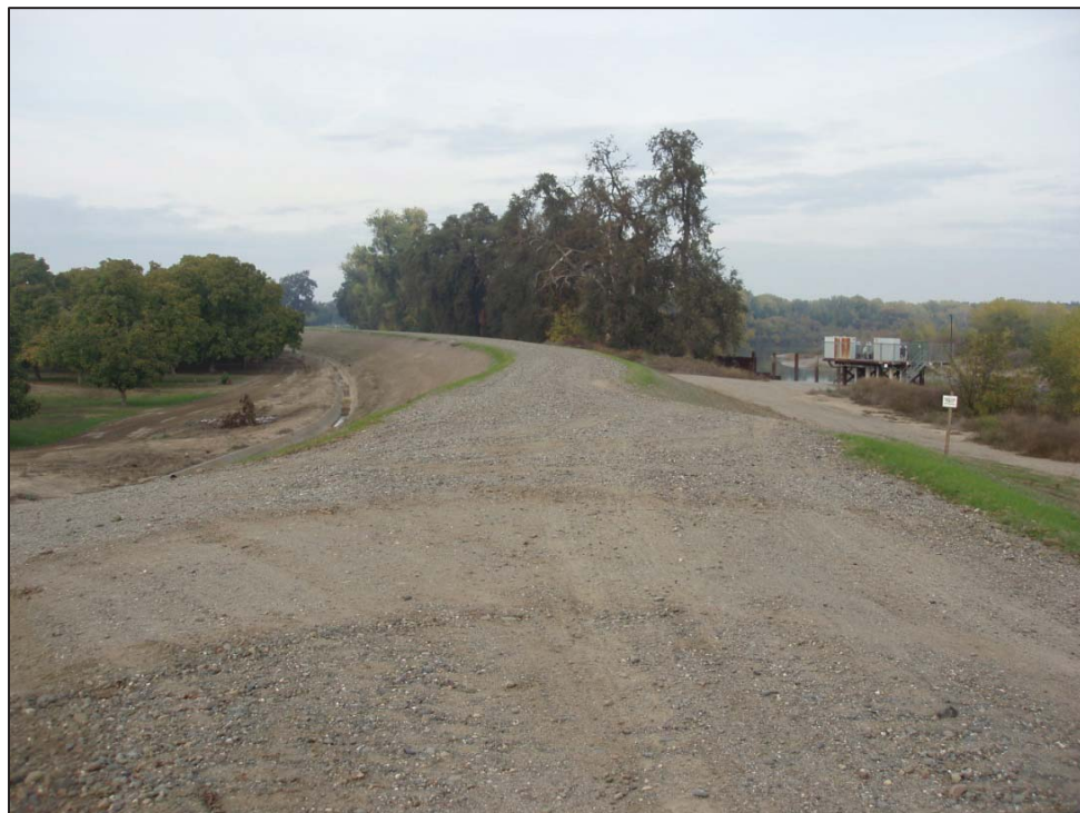
Figure 2: Maxwell Irrigation District, New pumphouse standing on the Sacramento River Levee, view looking north (C. Jimenez, November 13, 2012).
