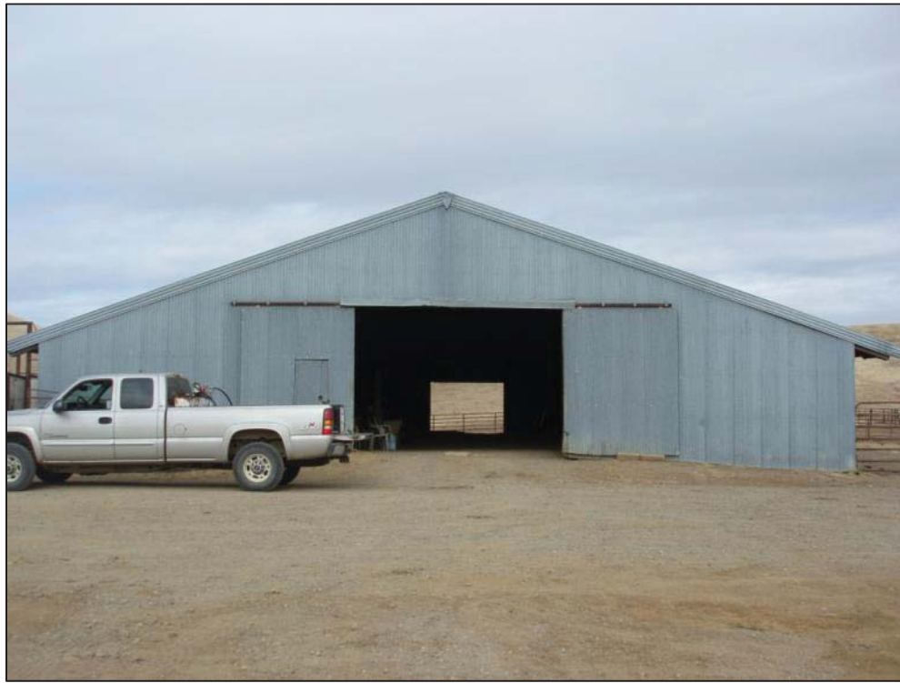
Figure 29: Edward Owens Farmstead, Lambing barn, view looking north (C. Jimenez, November 13, 2012).
