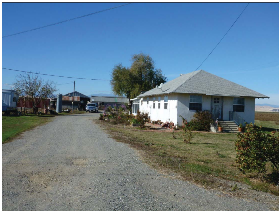
Figure 6: 4799 McDermott Road, House and Outbuildings, view looking west (C. Jimenez, November 14, 2012).
