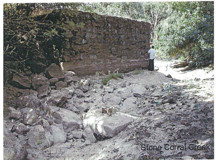
Photo 25: Feature 5, Footing and Western Bridge Abutment, Looking 210 Degrees E/N
