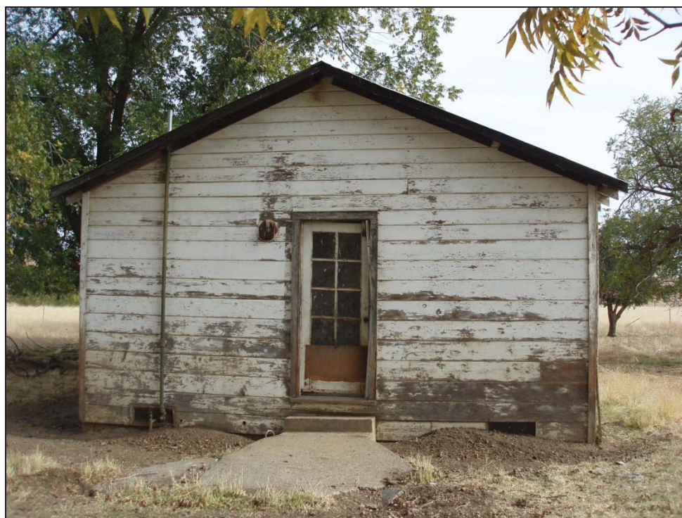
Figure 2: Shirley Jensen Farmstead, House, view looking east (C. Jimenez, November 13, 2012).
