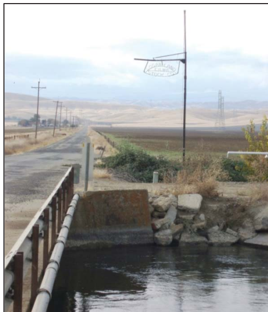
Glenn-Colusa Canal, looking west at County Road 68 (C. Jimenez 2012).
