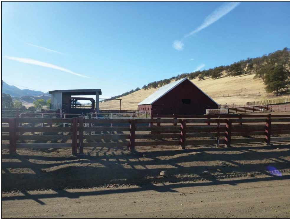
Figure 7: 3383 Huffmaster Road, barn and outbuilding, view looking southwest (C. Jimenez, November 14, 2012).
