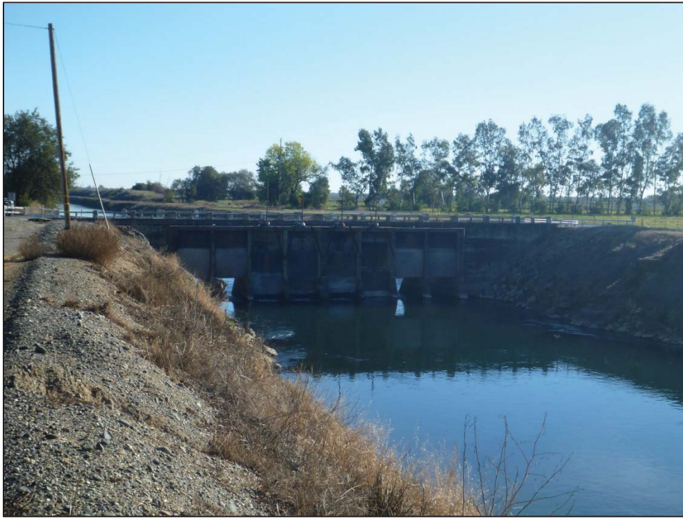
Figure 8: GCID Headgate, view looking southwest (C. Jimenez, November 14, 2012).
