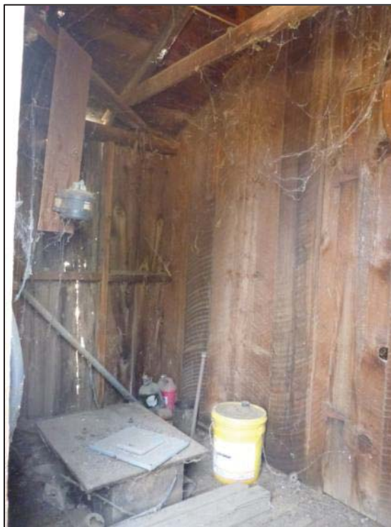
Figure 10: Edward Owens Farmstead, Shed B, interior detail (C. Jimenez, November 13, 2012).
