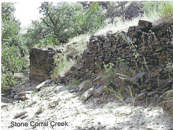
Photo 23: Feature 5, Retaining Wall and Bridge Abutment, Looking 52 Degrees E/N
