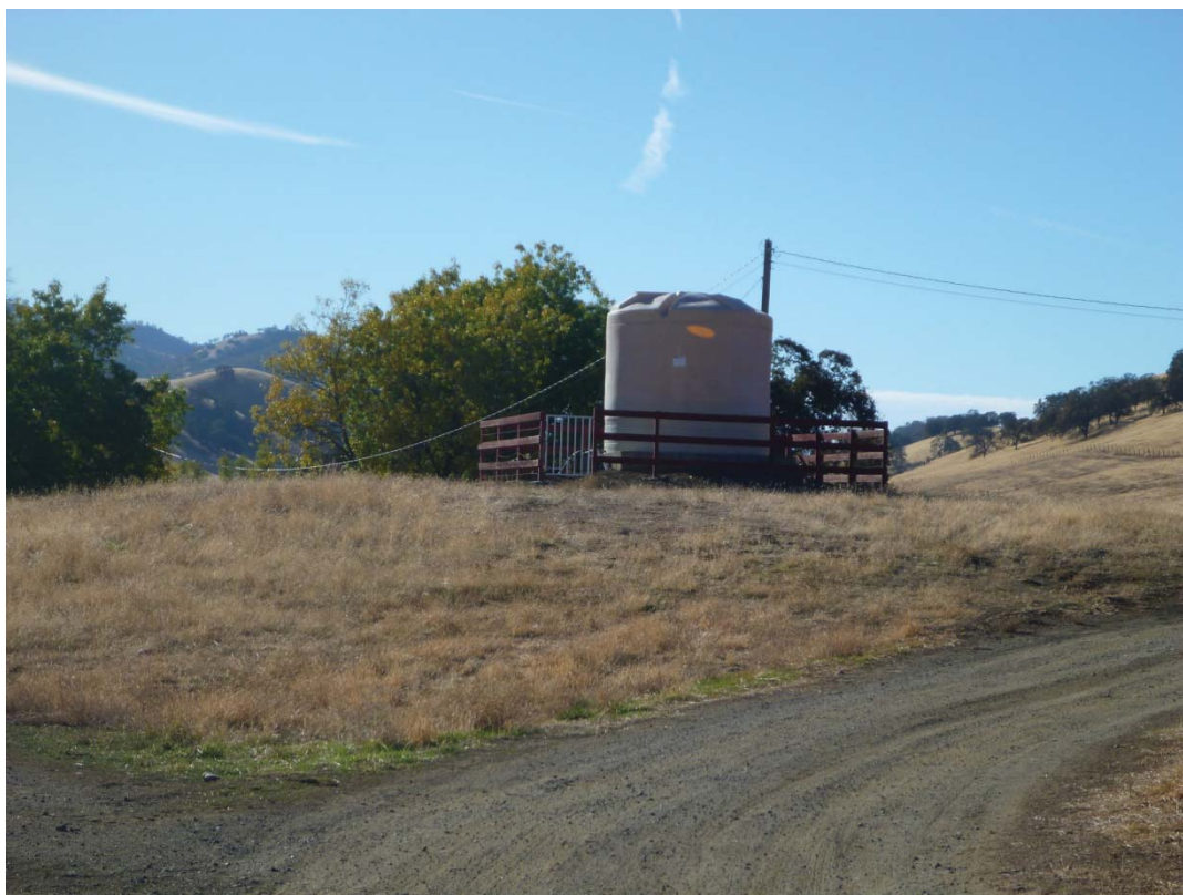
Figure 11: 3383 Huffmaster Road, water tower, view looking south (C. Jimenez, November 14, 2012).
