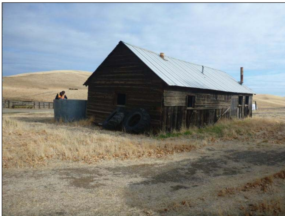
Figure 12: Edward Owens Farmstead, Bunkhouse, view looking northeast (C. Jimenez, November 13, 2012).
