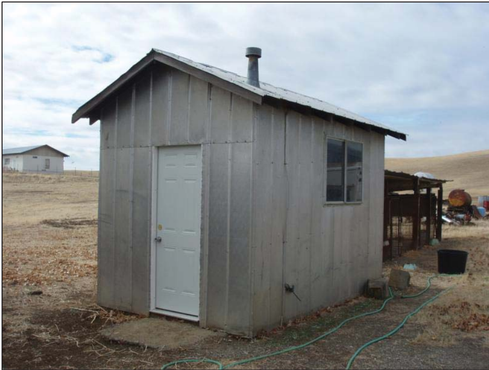
Figure 21: Edward Owens Farmstead, Metal shed, view looking west (C. Jimenez, November 13, 2012).
