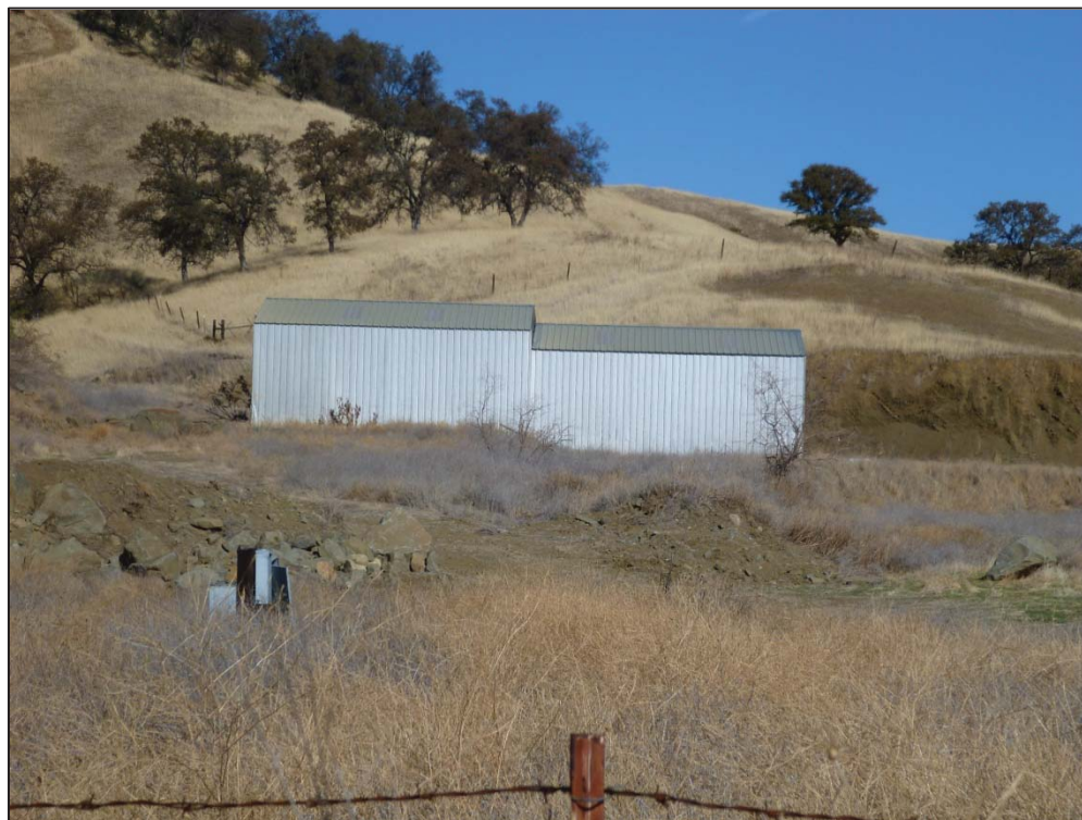
Figure 10: Knowles Quarry, outbuilding, view looking north (C. Jimenez, November 14, 2012).
