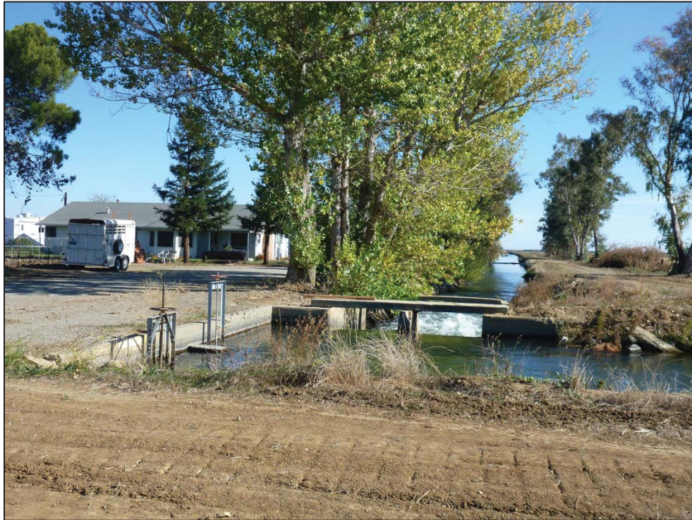
Figure 5: 4790-92 McDermott Road, House and irrigation canal, view looking east (C. Jimenez, November 14, 2012).
