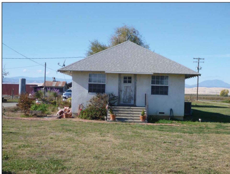
Figure 5: 4799 McDermott Road, House, view looking west (C. Jimenez, November 14, 2012).
