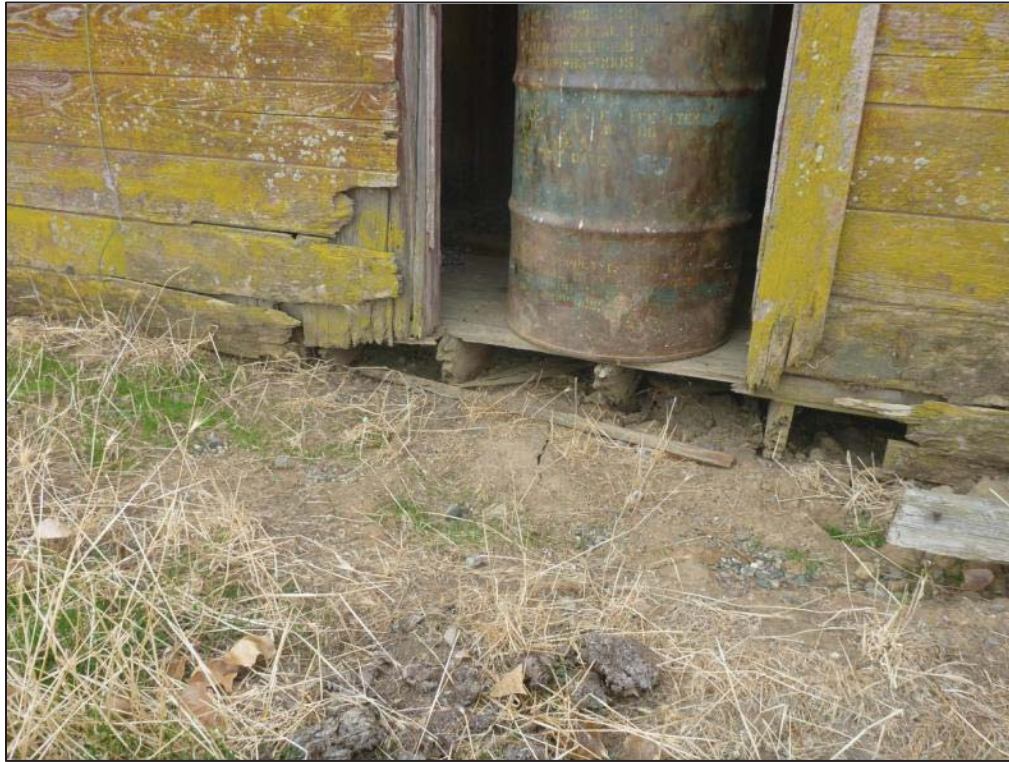
Figure 13: Edward Owens Farmstead, Bunkhouse, foundation detail (C. Jimenez, November 13, 2012).
