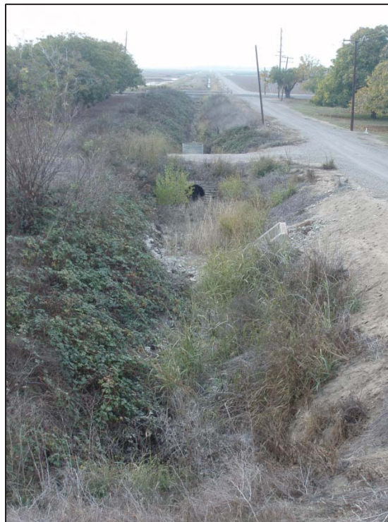
Figure 14: Maxwell Irrigation District, Abandoned canal, view looking west (C. Jimenez, November 13, 2012).
