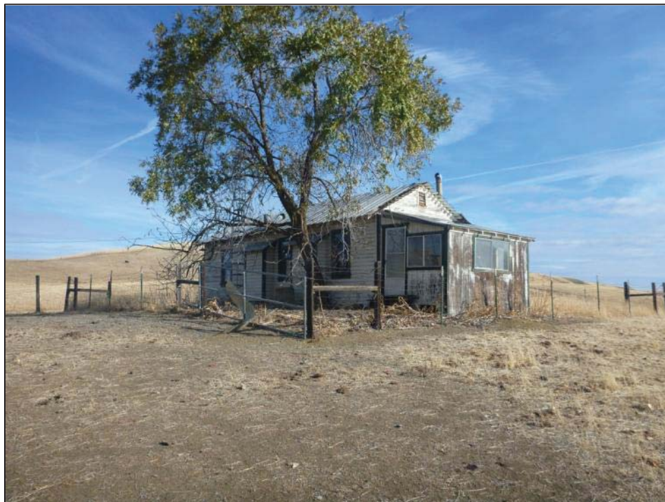
Figure 4: Edward Owens Farmstead, House, view looking northeast (C. Jimenez, November 13, 2012).
