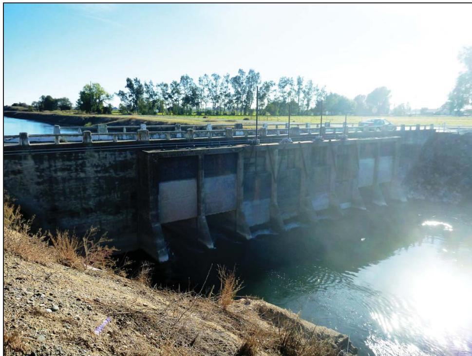
Figure 9: GCID Headgate, north elevation (C. Jimenez, November 14, 2012). (Note, 8 valve openings on gate).
