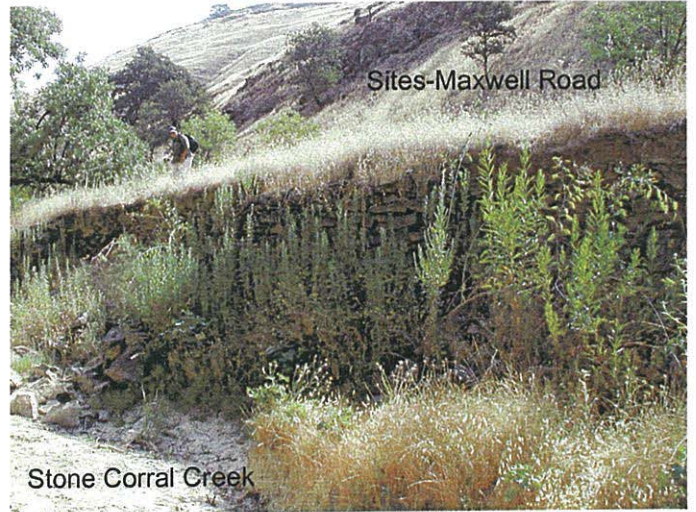
Photo 22: Feature 5, Retaining Wall, Looking 70 Degrees E/N
