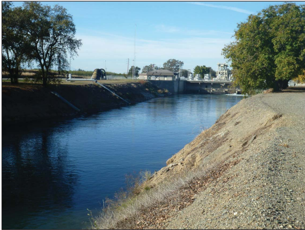
Figure 6: GCID 1983 Pumping plant and canal prism, view looking northwest (C. Jimenez, November 14, 2012).
