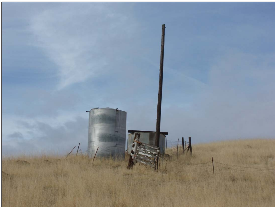
Figure 16: Shirley Jensen Farmstead, Water tank and possibly pumphouse, view looking west (C. Jimenez, November 13, 2012).
