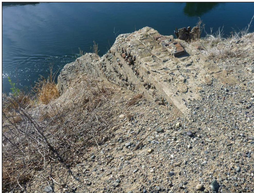
Figure 11: GCID remains of historic headgate (C. Jimenez, November 14, 2012).
