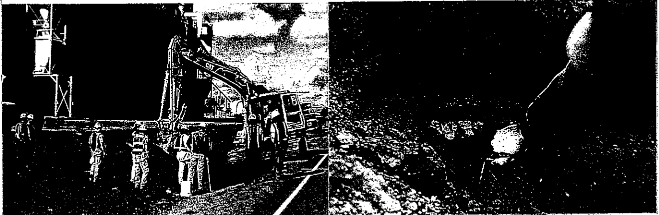
Figure 35: Left - Excavating Trench 38 alongside Stegeman Station; Right - House floor found in Trench 33, 3.0' below surface.
