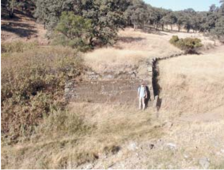
Figure 48: SF-038-A, CLRR south abutment and retaining wall.
