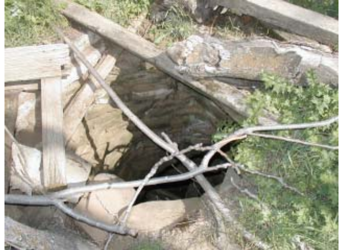
Figure 43: Open, stone lined well located at the historical site on the Alfred A. Shearin Sale-Cash Entry property.
