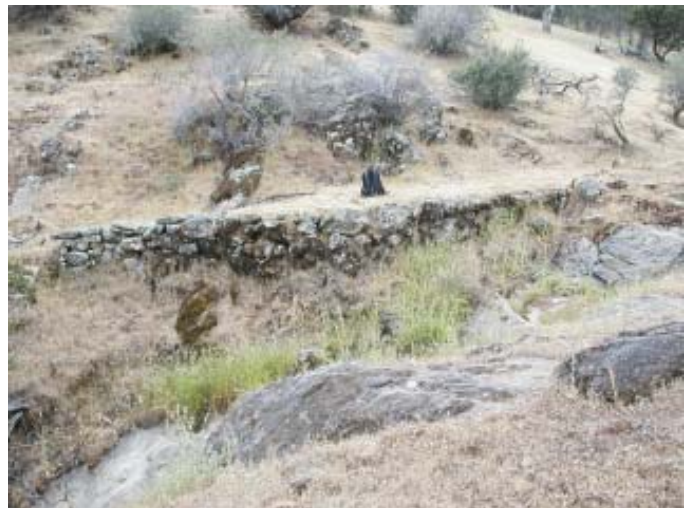
Figure 47: Isolate SF-ISO-008-C, streamside retaining wall along the old Sites-Lodoga Road.
