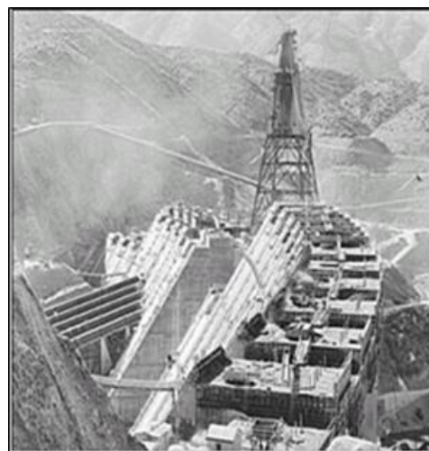
Shasta Dam Under Construction
