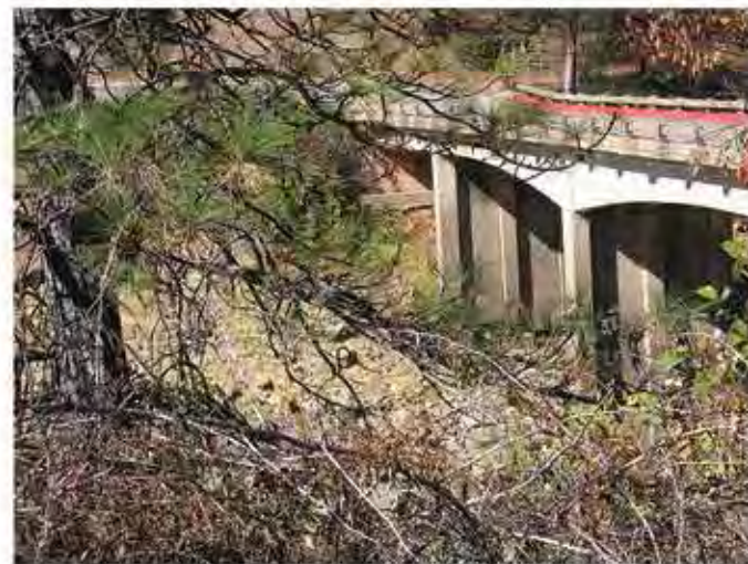
McCloud Arm VAU, KOP 16, Photo 16 View of the McCloud River Bridge, from the eastern approach.
