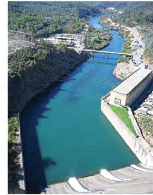
Shasta Dam VAU, KOP 2, Photo 2b View of the Shasta Dam spillway and the upper Sacramento River from Shasta Dam.
