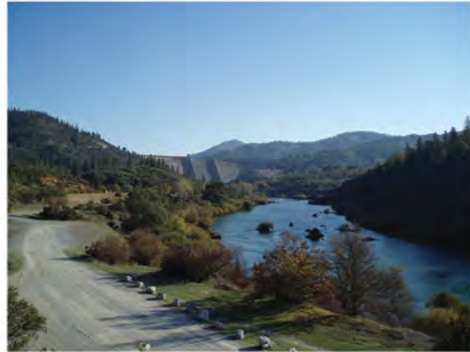
Shasta Dam VAU, KOP 9, Photo 9a View from the road above the Chappie - Shasta OHV Area staging area looking northeast.
