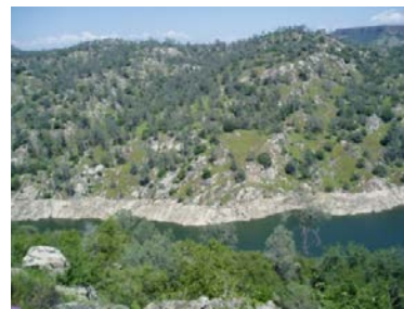
View of Temperance Flat RM 274 dam site from top of left abutment
