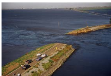
Jones Tract Levee Failure, 2004 Source: California Department of Water Resources
