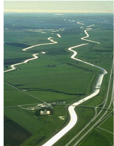
Delta-Mendota Canal and California Aqueduct
