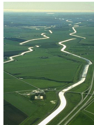
Delta-Mendota Canal and California Aqueduct
