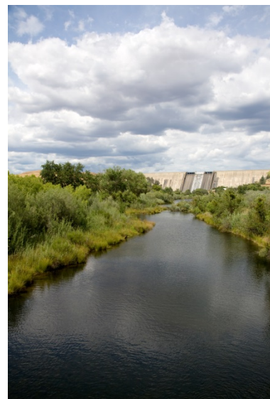
San Joaquin River and Friant Dam
