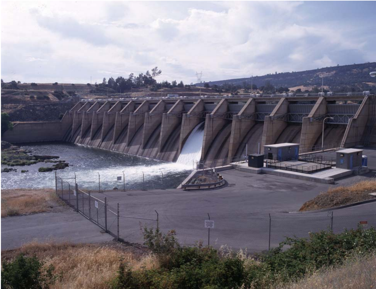
Figure A.2.1-4. Thermalito Diversion Dam and the Thermalito Diversion Dam Powerplant.
