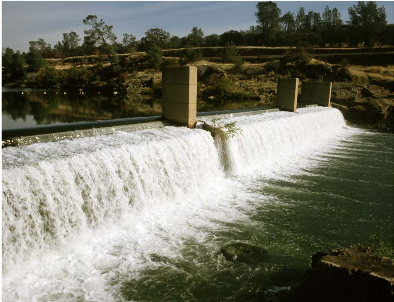
Figure A.2.2-1. Fish Barrier Dam.
