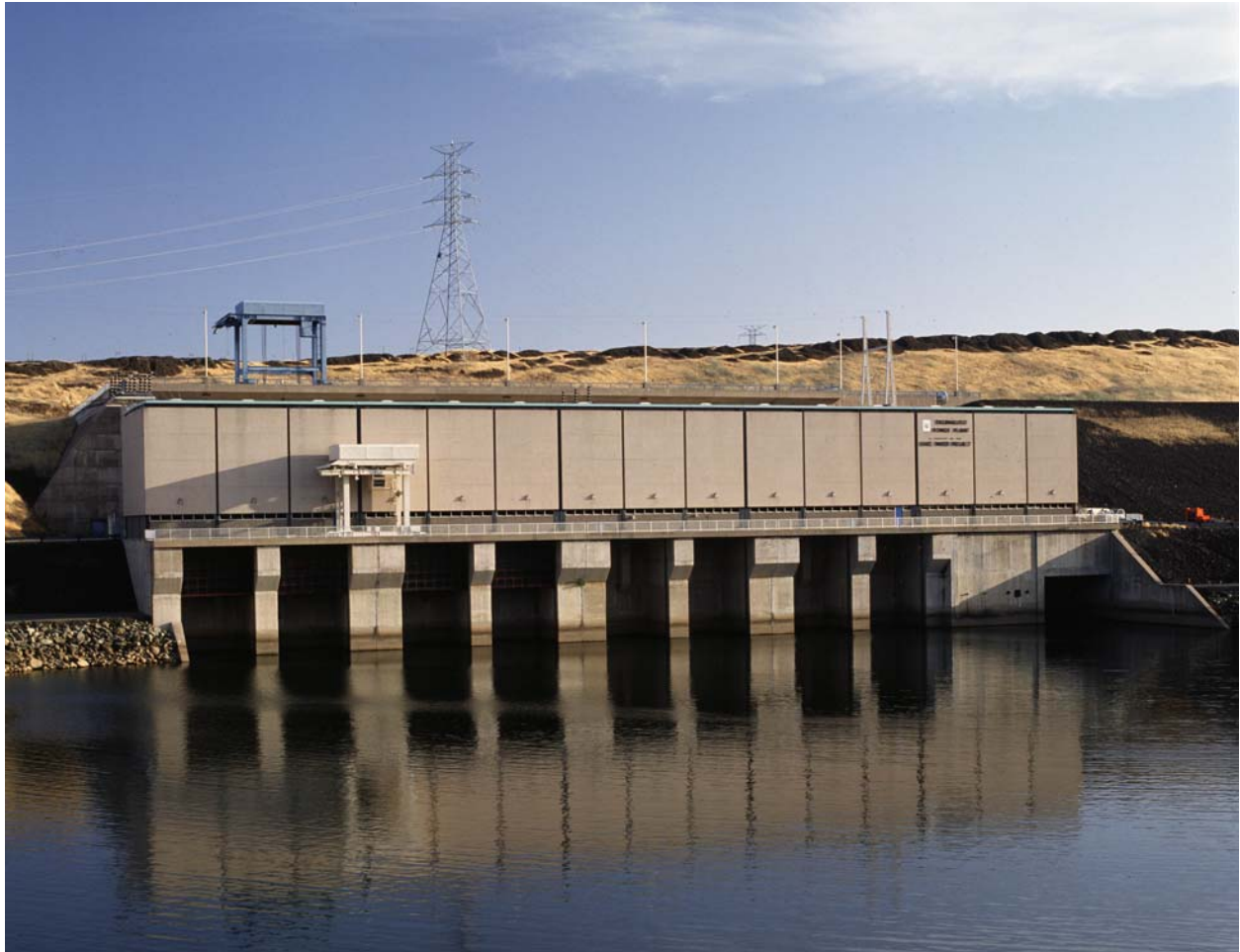
Figure A.2.1-7. Thermalito Pumping-Generating Plant.
