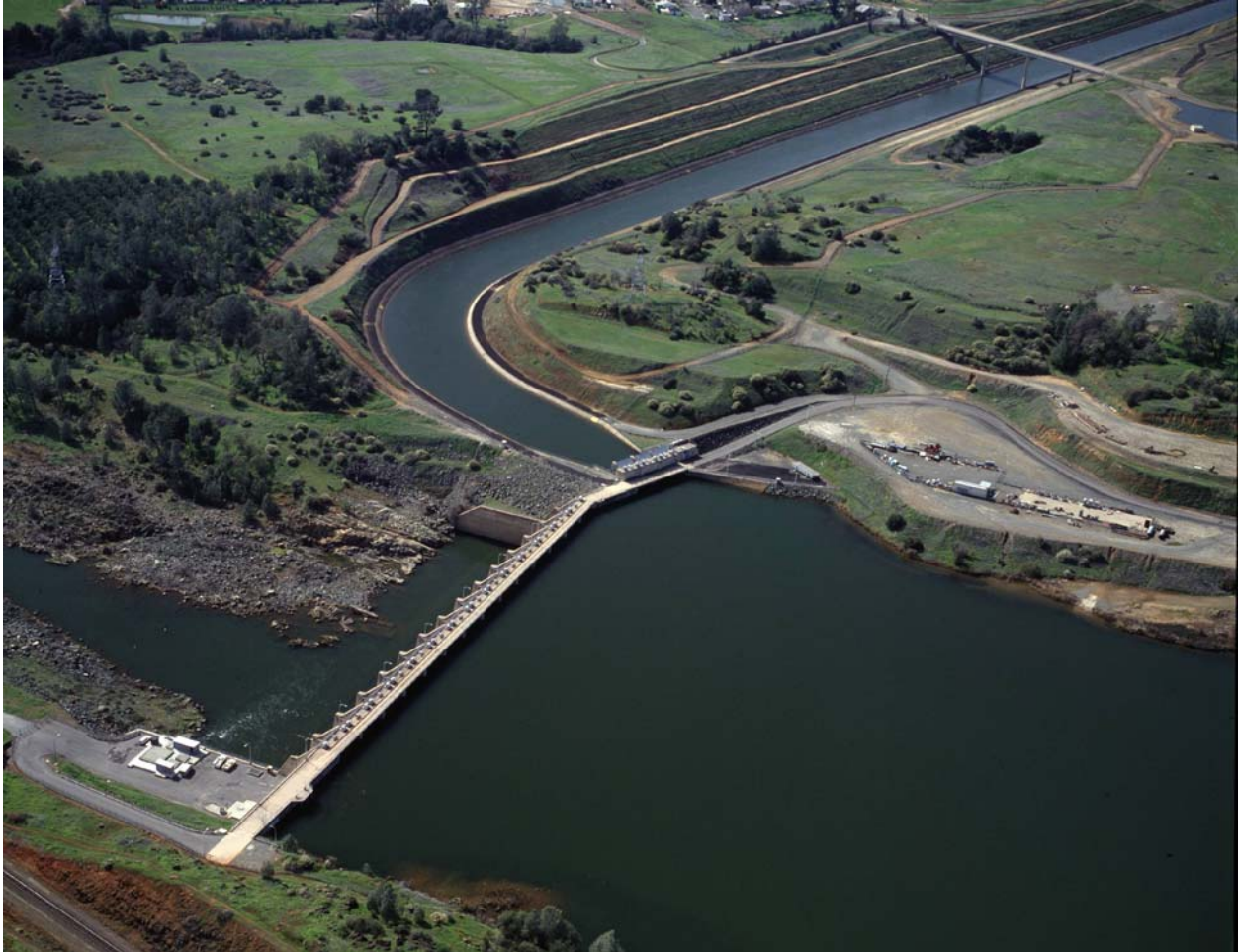
Figure A.2.1-5. Thermalito Diversion Dam and the Thermalito Power Canal.
