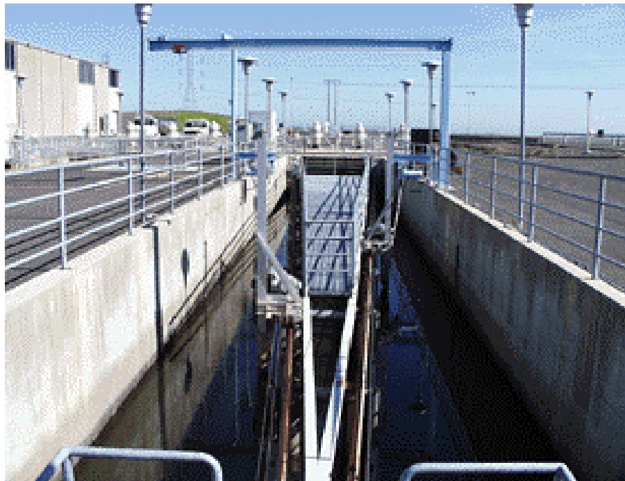
Photograph J-6. Close-Up View of the Skinner Fish Facility Secondary Louver Channels Channels divert fish on their way to the sampling area. (Source: California Department of Water Resources; Photograph by Steve Foss, California Department of Fish and Game.)
