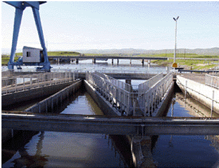
Photograph J-5. Close-Up View of the Skinner Fish Facility Primary Louver Channels Diversion bays direct fish toward secondary channels. (Source: California Department of Water Resources; Photograph by Steve Foss, California Department of Fish and Game.)
