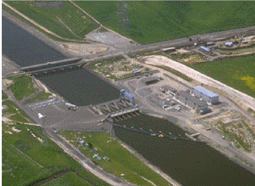
Photograph J-3. Aerial View of the John E. Skinner Fish Facility in Byron, California Located between Clifton Court Forebay and the SWP Banks Pumping Plant. (Source: California Department of Water Resources.)
