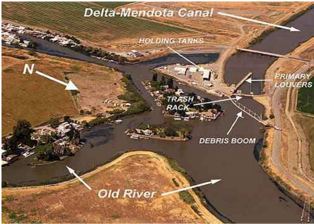
Photograph J-1. Aerial View of the CVP Tracy Fish Facility on Old River at the Entrance to the Delta-Mendota Canal Intake Channel Leading to the CVP Tracy Pumping Plant (Source: Bureau of Reclamation.)
