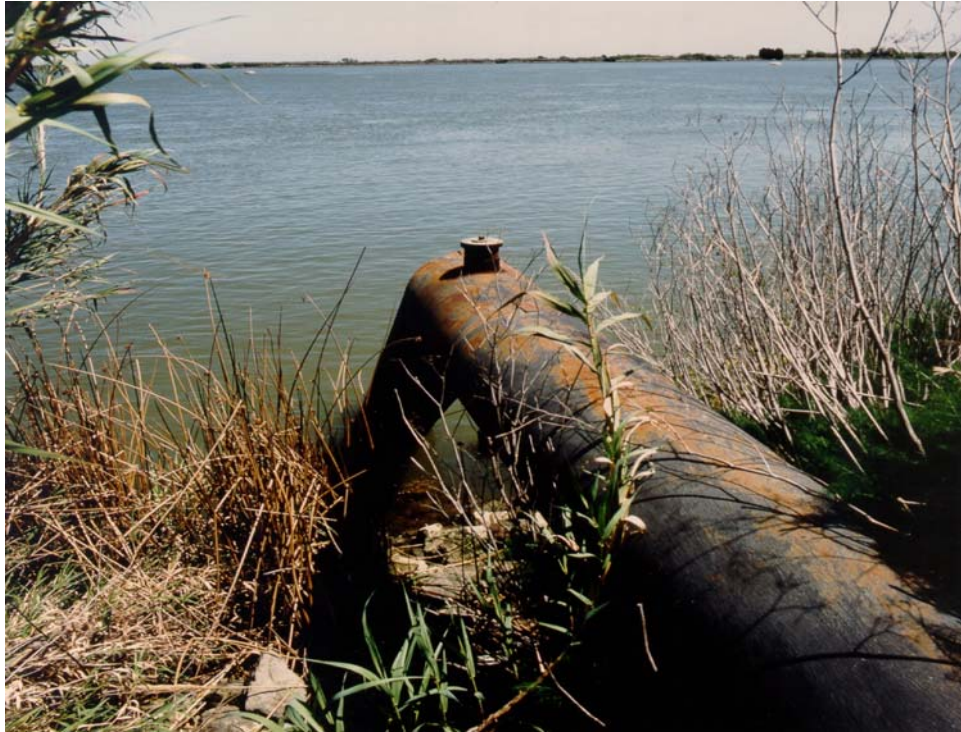
Photograph 5.3-9. Agricultural Diversion Siphon That Supplies Irrigation Water from the Delta Channels (Source: California Department of Water Resources.)
