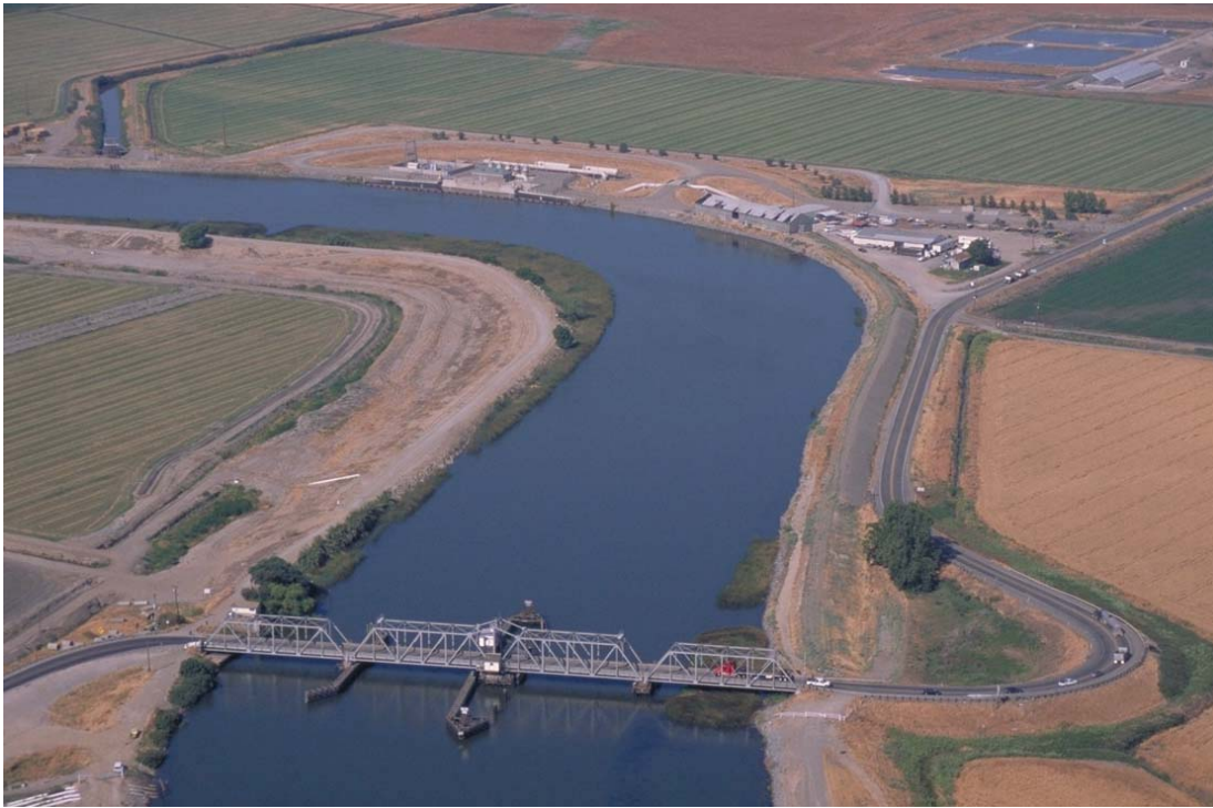
Photograph 5.3-11. Los Vaqueros Intake Located on the Western Bank of Old River Just Upstream (South) of the State Route 4 Bridge (Source: California Department of Water Resources.)
