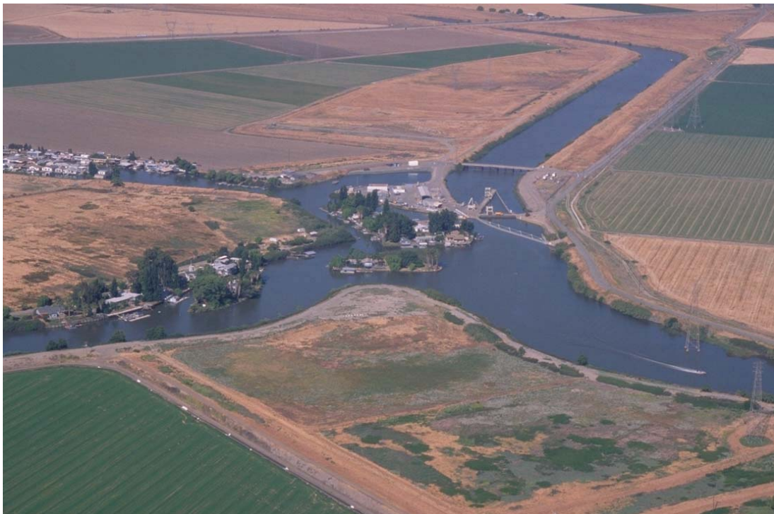
Photograph 5.3-14. Intake to the Central Valley Project Delta-Mendota Canal Located just Upstream (South) of Grant Line Canal (Source: California Department of Water Resources.)
