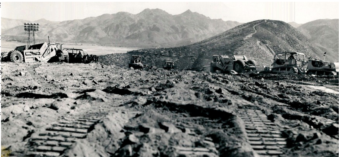
Above: Building the Cedar Springs Dam.
